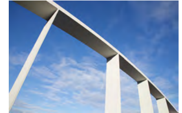
Painted Steel Structure
