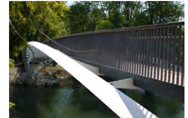
Painted Steel Parapet
