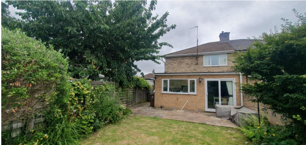
Rear garden elevation view
