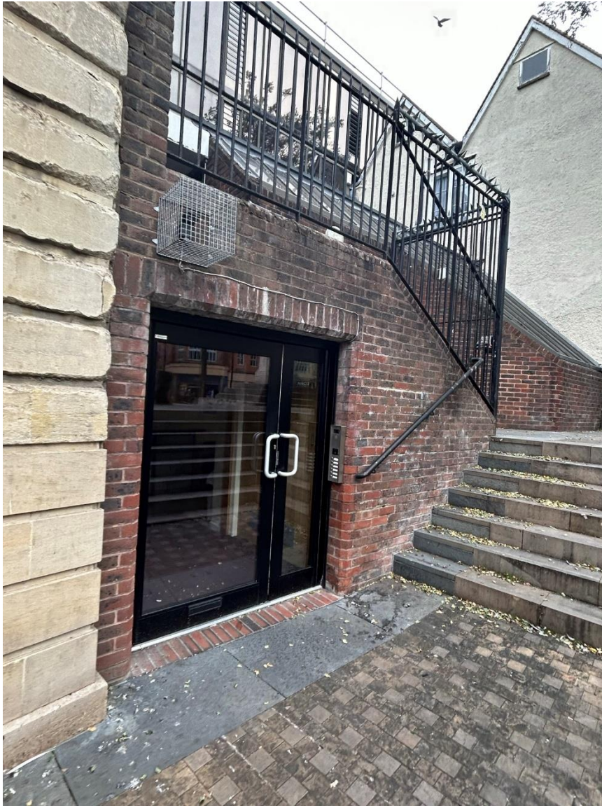
Close up photo of existing doorset.
