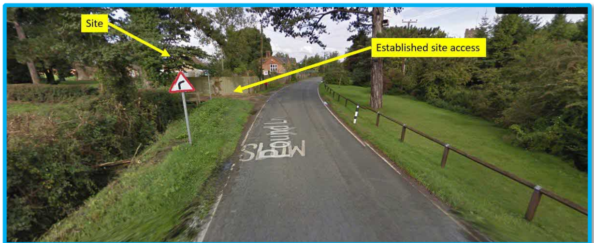
Figure 11 Goole Streetview image showing substantial roadside ditches, Pound Lane above the surrounding land and the established site access.
