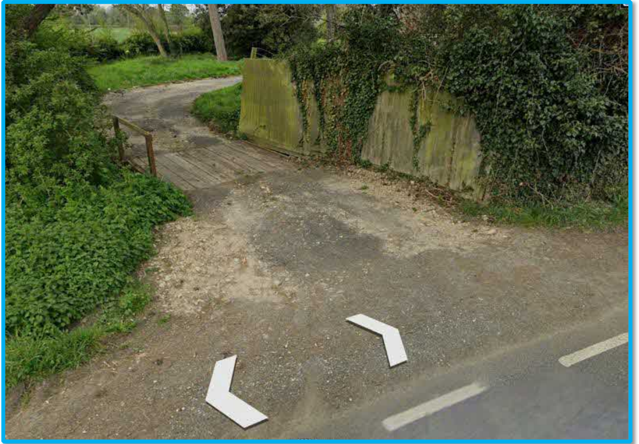
Figure 12 Established site access off Pound Lane
