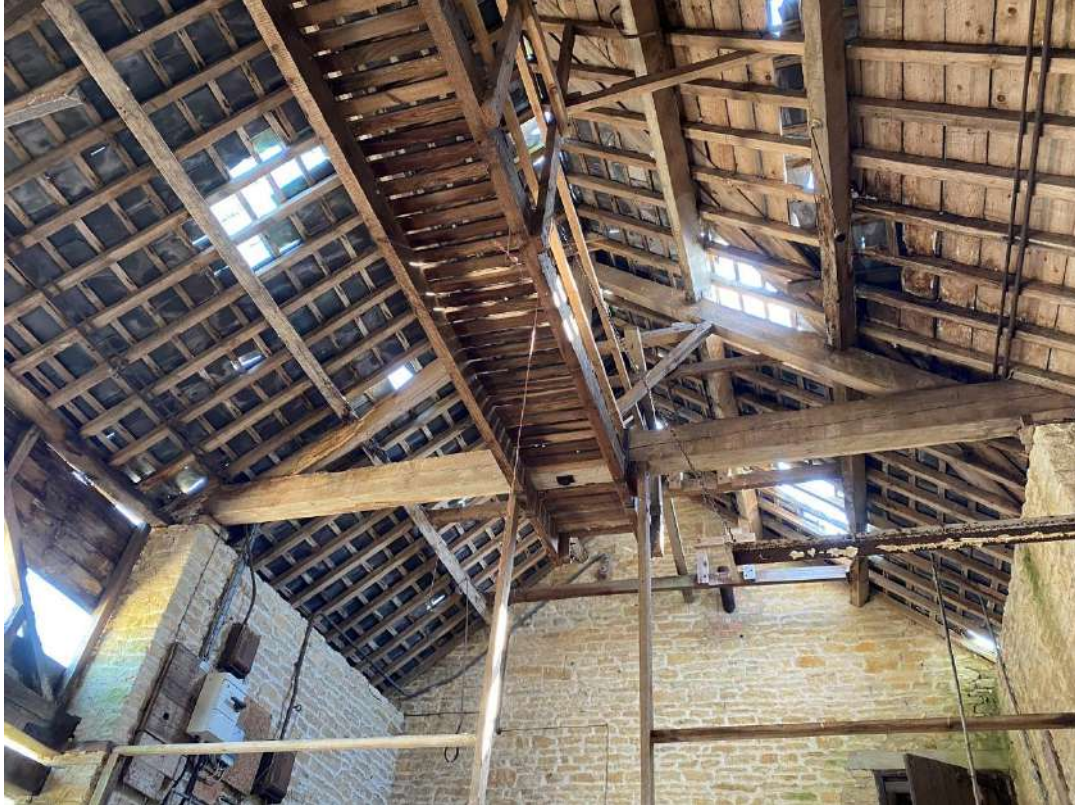
Figure 1 - Existing Roof Structure to Northern Half of Barn
