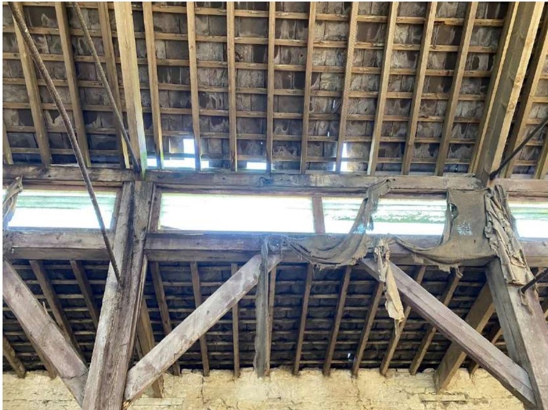
Figure 2 - Existing Roof Structure of Southern Half of Barn
