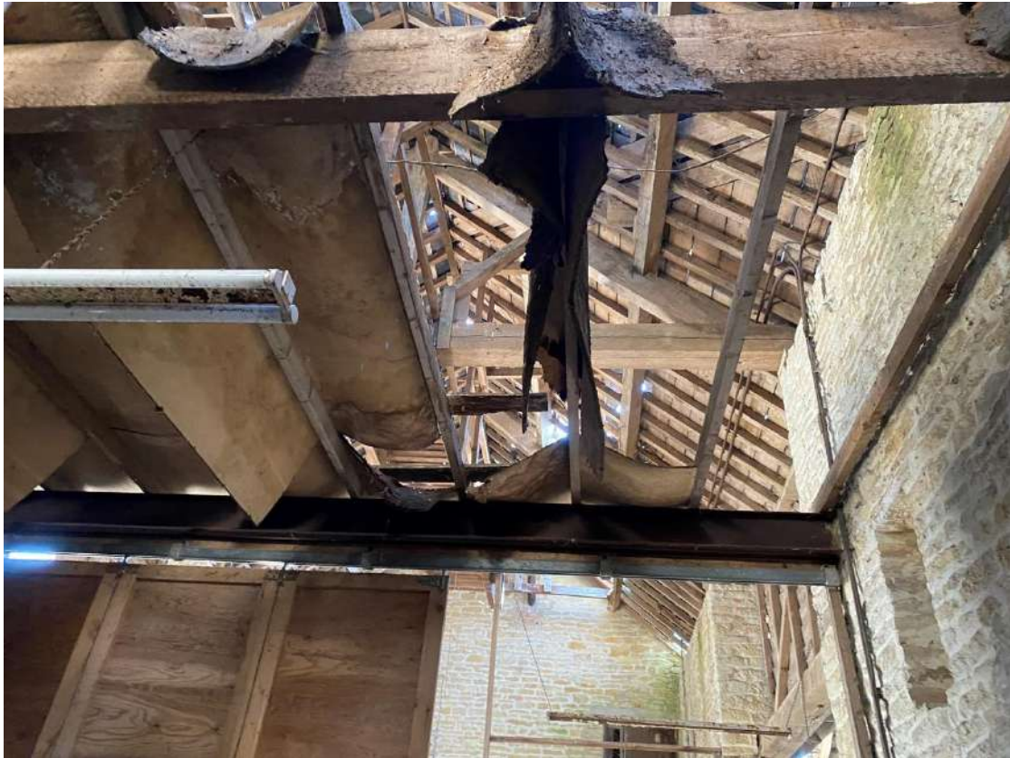
Figure 3 - Remains of Mezzanine Floors
