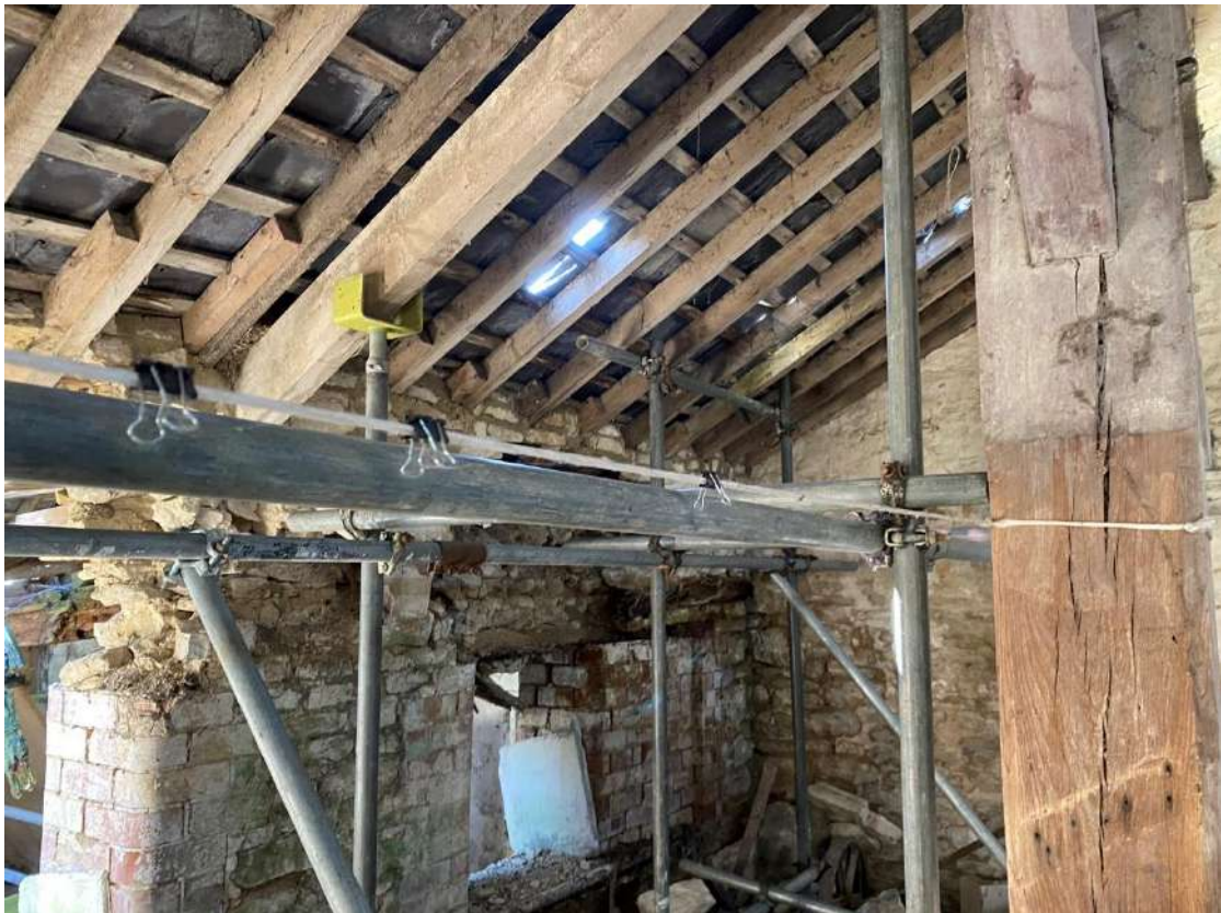
Figure 11 - Scaffold Support to Covered Yard Roof
