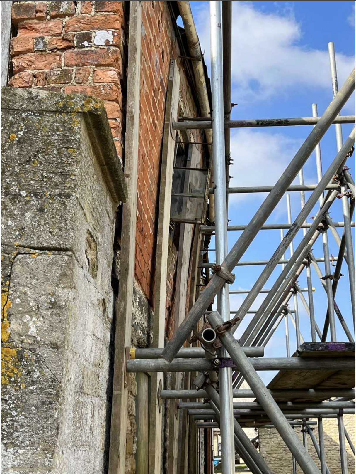
Figure 14 - Outward Movement of Roof and Northern Wall
