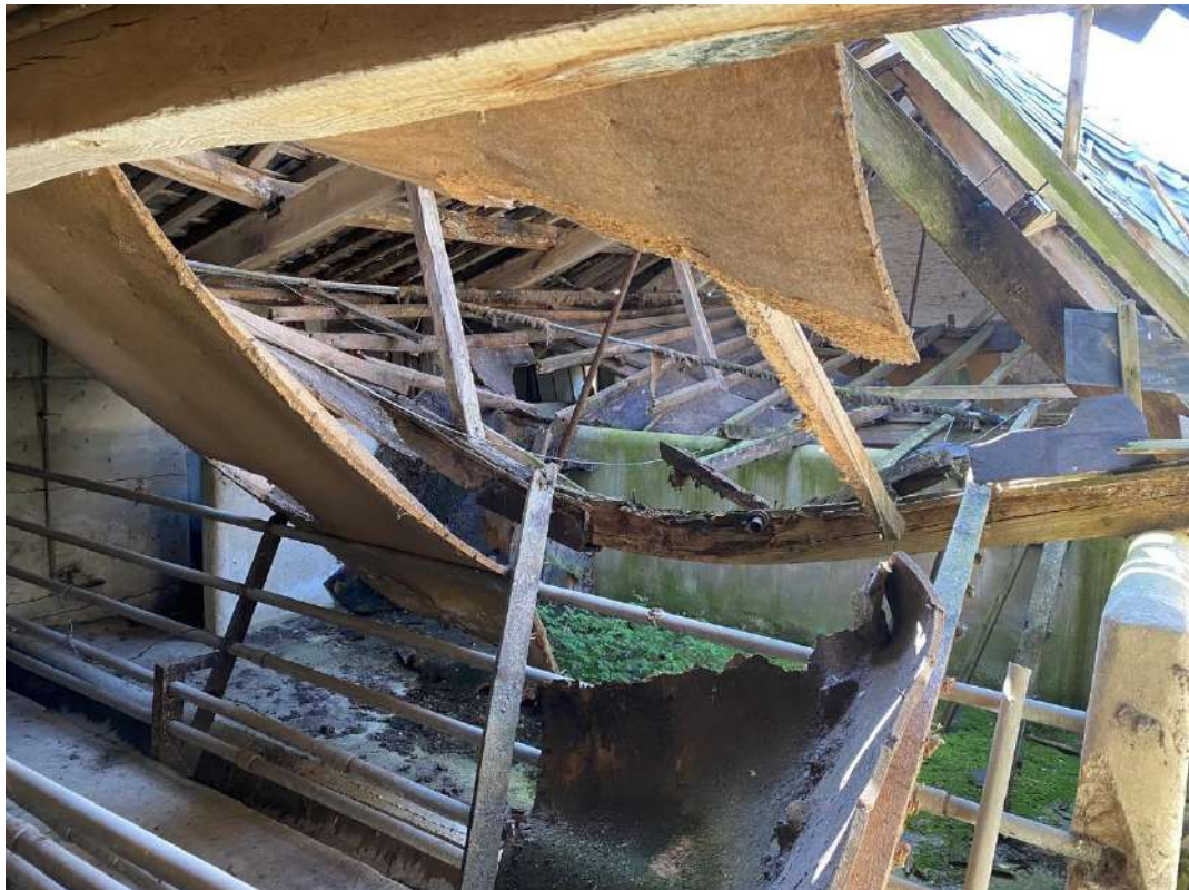
Figure 2 - Failed Truss
