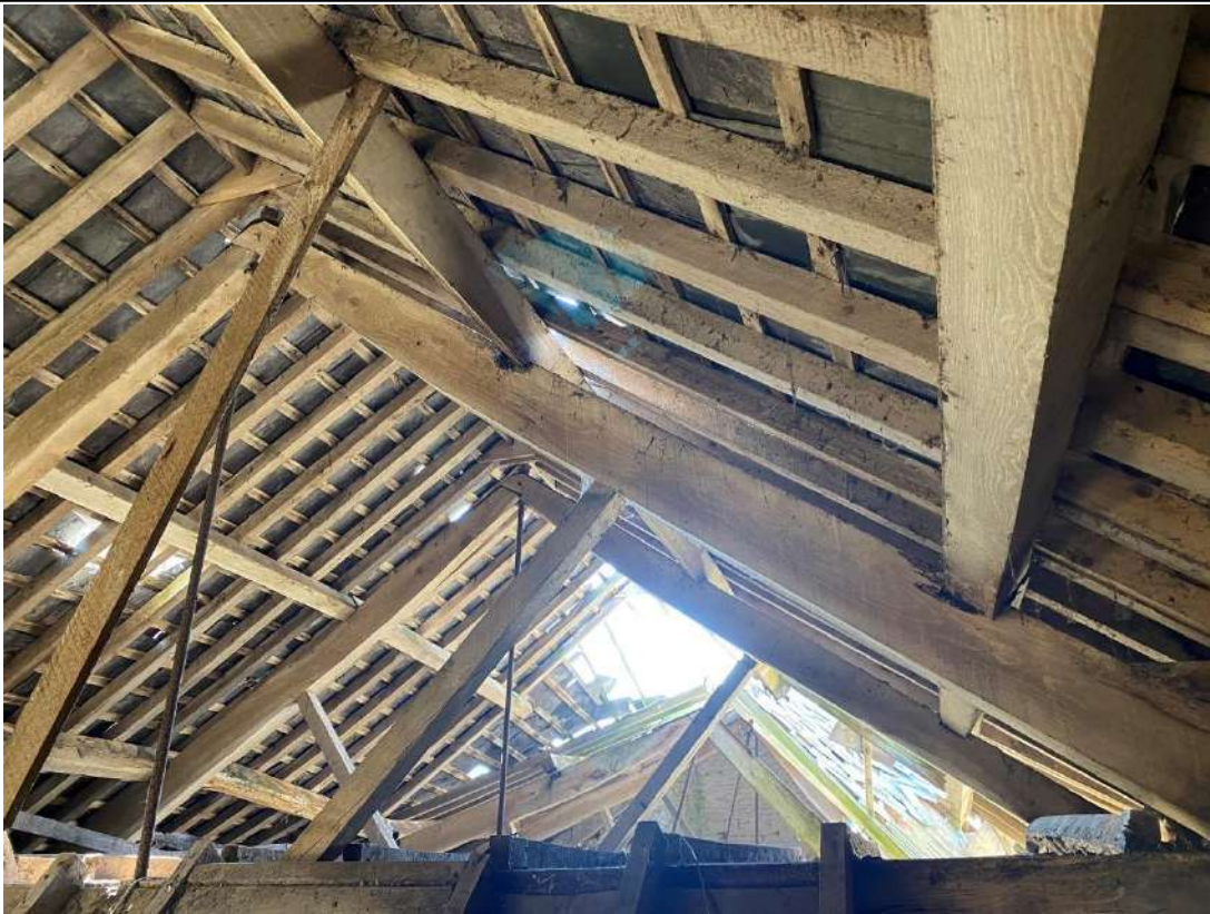
Figure 5 - Decay of Truss Rafter and Purlins at Bearing of Purlin onto Truss
