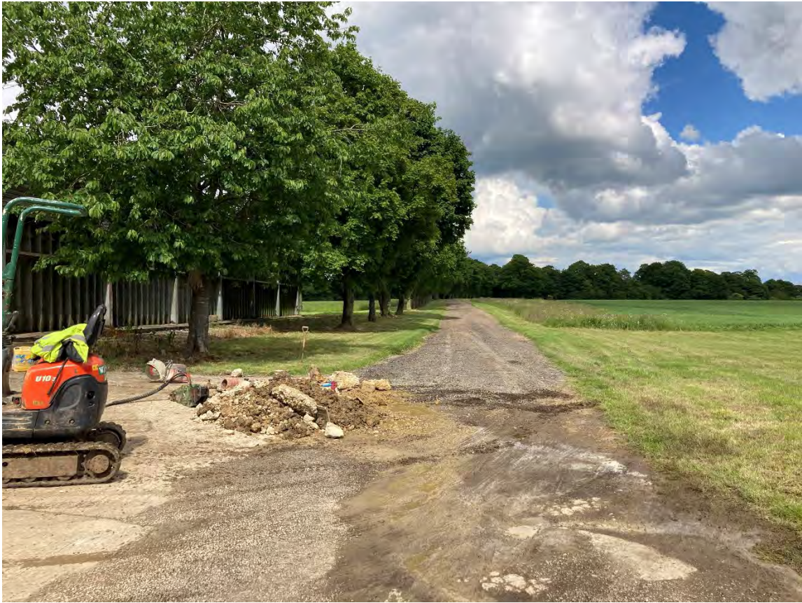
Plate 3: View from within Asterleigh Farm buildings, looking north-east along north-eastern access
