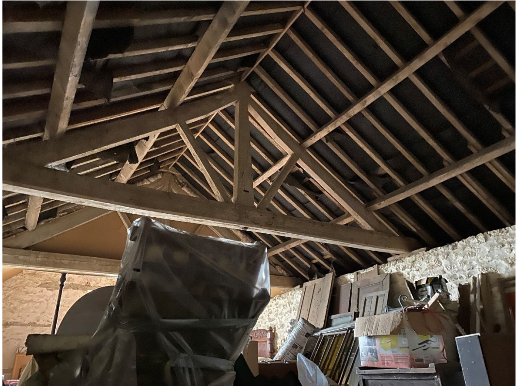
Figure 37: Roof structure in Building 7
