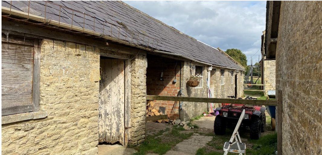
Figure 13: Building 1A, the northern range of stables.
