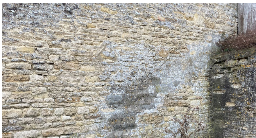
Figure 21: blocked triangular ventilation hole in the northern elevation of Barn 2B with scar from removed tallet steps beneath.
