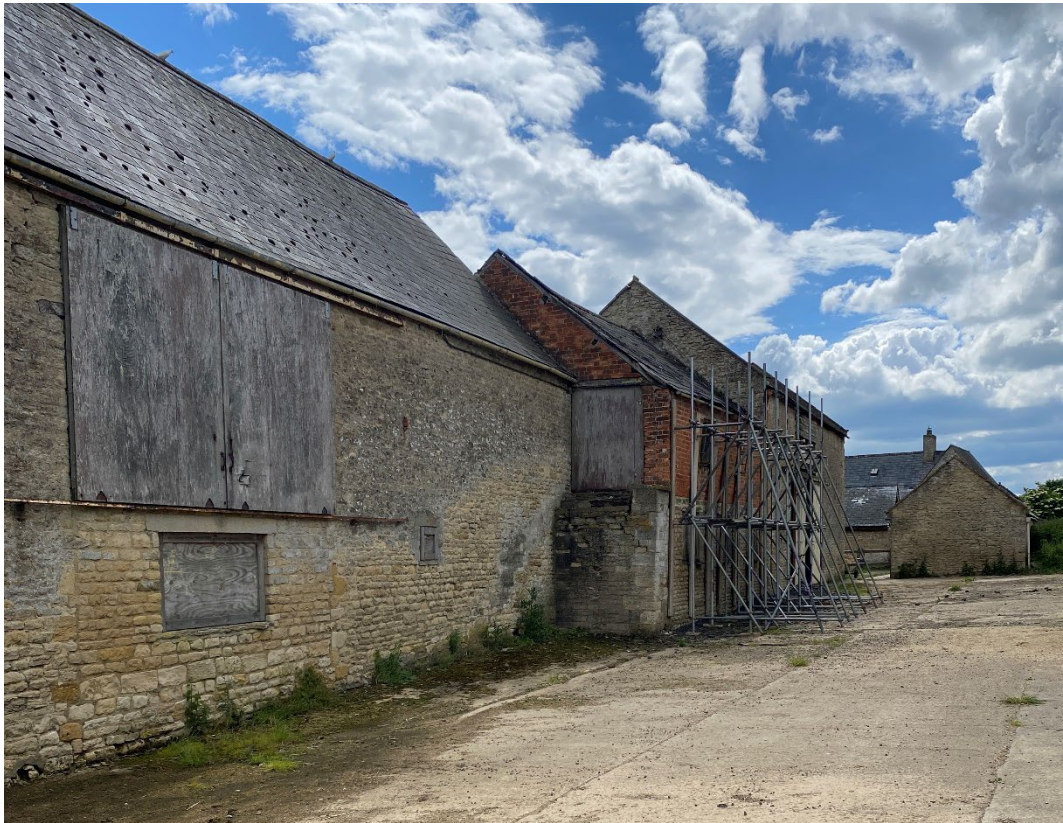
Figure 18: View along the northern edge of Building 2 looking towards the chimney and roof of the farmhouse and gable end of Building 1, the left hand structure is earlier, the far right one a later addition with later infilling structure in red brick.
