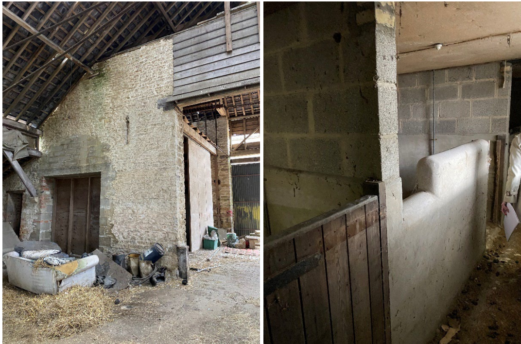
Figures 24-25: (Left the south western elevation of the threshing barn 2A with inserted opening and narrow 'candle' ventilation slit and, (right) concrete block subdivisions in the lower part of the linking structure.
