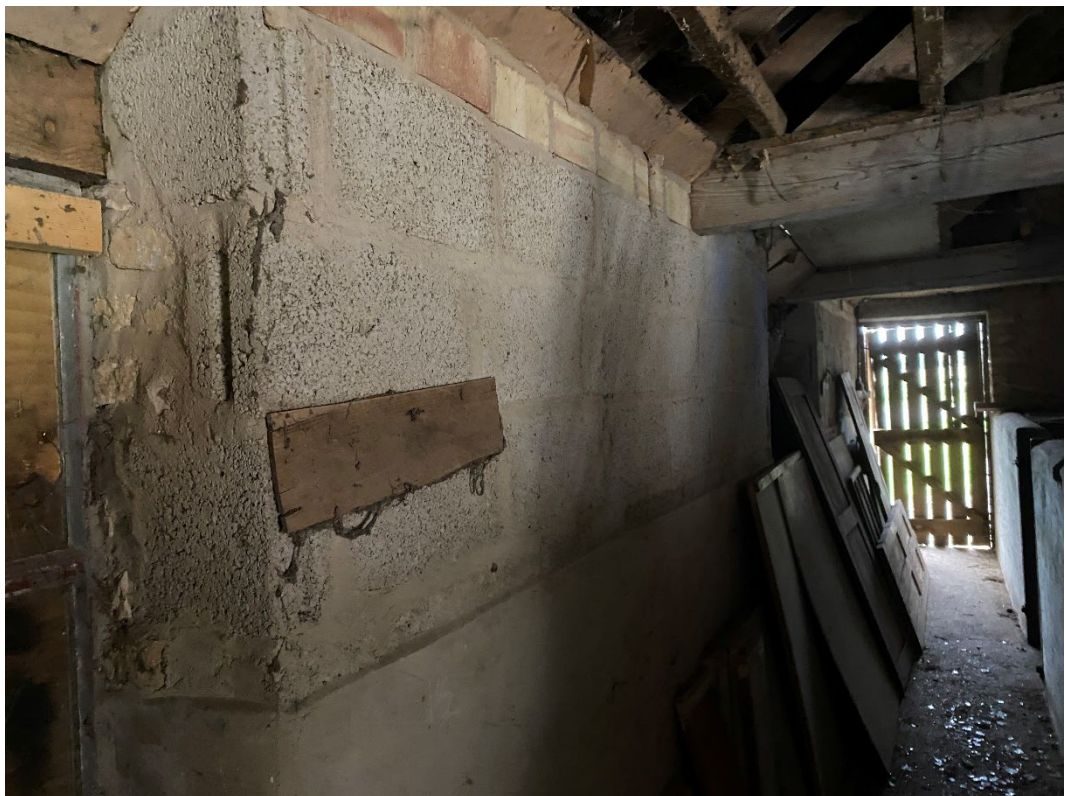
Figure 35: concrete blockwork internally within Building 6.
