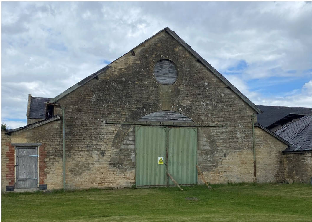
Figure 30: Building 4, southern façade, infilled arched opening and blocked roundel window. The vertical portions to either side are louvered along the long elevations.
