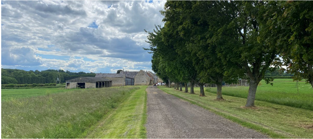
Figure 42: The approach to Asterleigh Farm from the east. The modern barn (Building 8) to the southeast is most prominent and the farmhouse is not visible at all.
