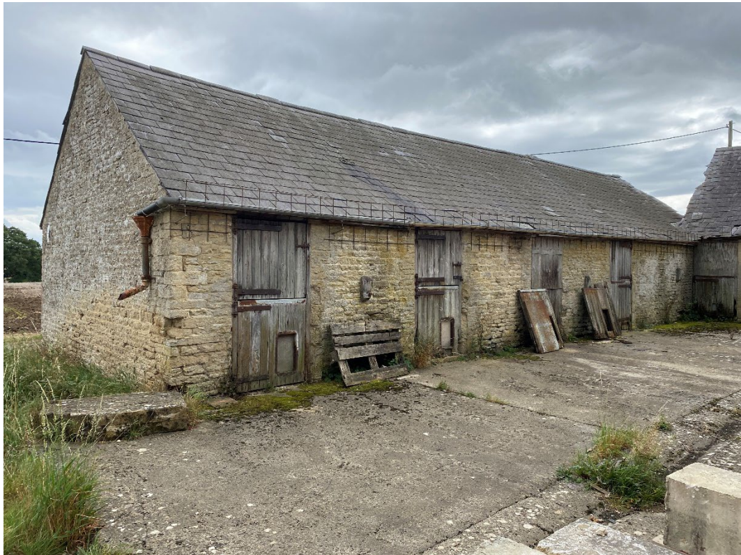
Figure 33: Barn 6 though on an historic footprint apparently a much later reconstruction.
