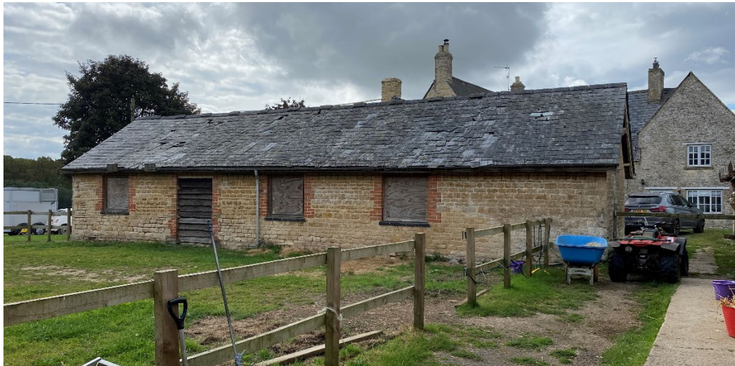
Figure 15: Building 1B: the western stable, a later addition.
