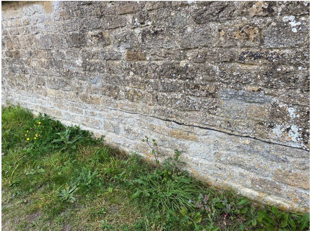
Figure 34: Rear wall of Building 6 with visible DPC
