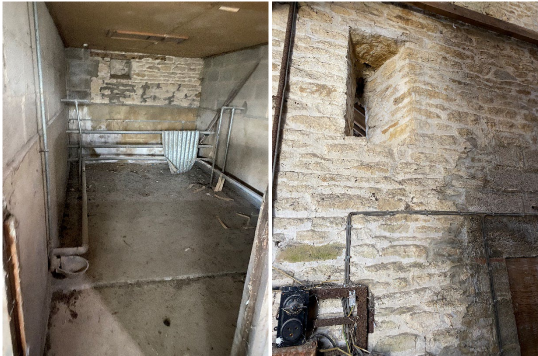
Figure 48-49: Pigsties to be removed, block work partitions, galvanised manger, note blocked window cut across by stall divider on left of image; (right) narrow 'candle' opening in threshing barn to glaze internally and replicate/reinststate where blocked.
