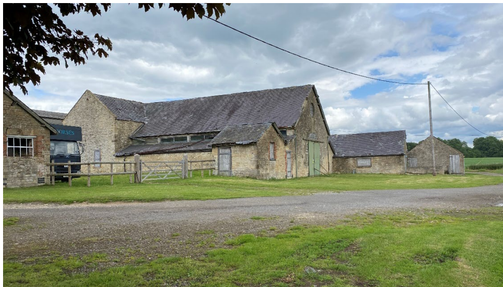
Figure 30: Barn 4 currently filling the central of the historic open yards and the southern elevation of the 18 th century Barn 2 from the south.
