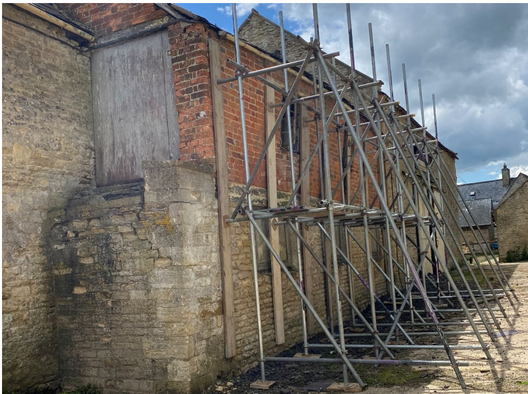
Figure 47: The central linking structure between threshing barns to become part of Plot 2, featuring extant window openings that can simply be reused, including the former hay loft door, now missing its external steps.
