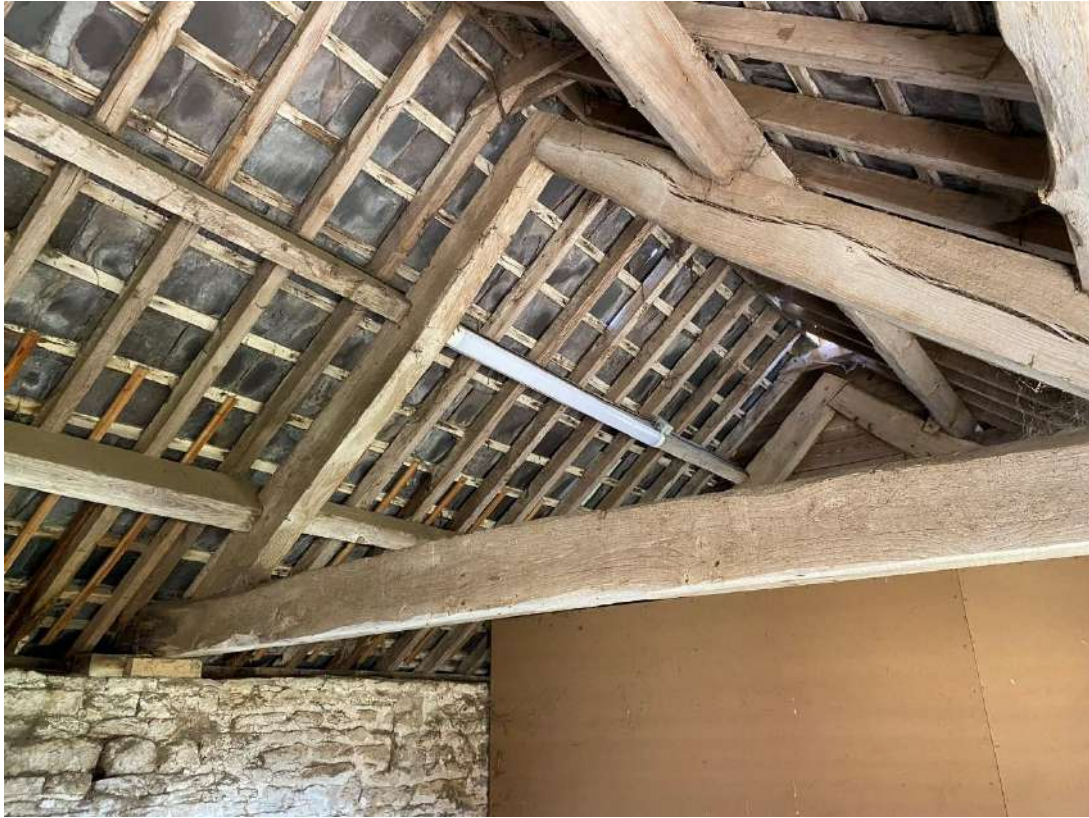
Figure 1 - View of Stable Roof
