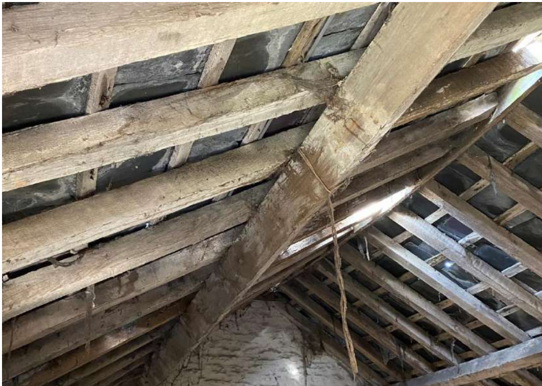
Figure 2 - View of Storeroom Roof
