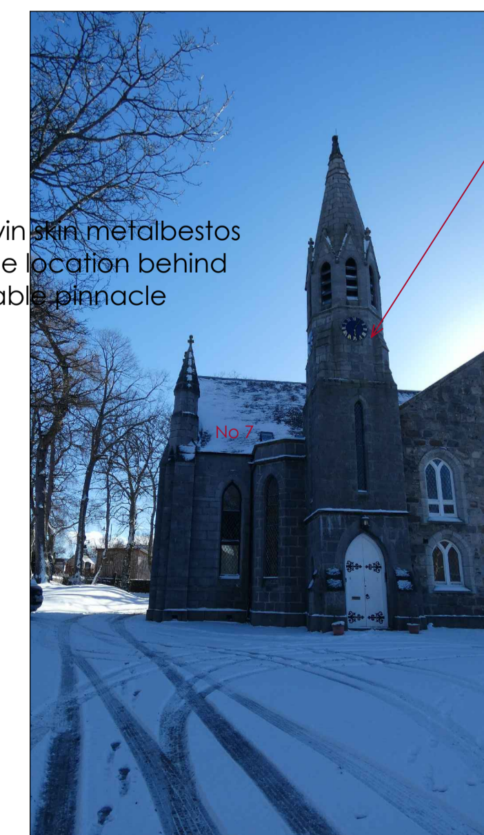
Cluniebank Gardens - North elevation
