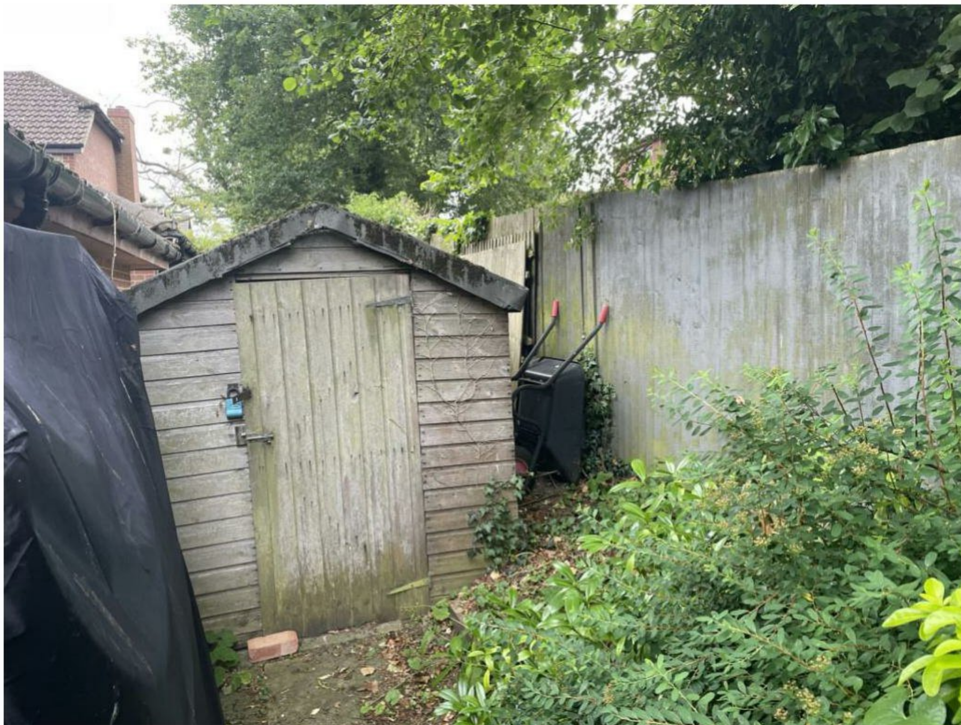
Shed to be moved and reinstated by others.
