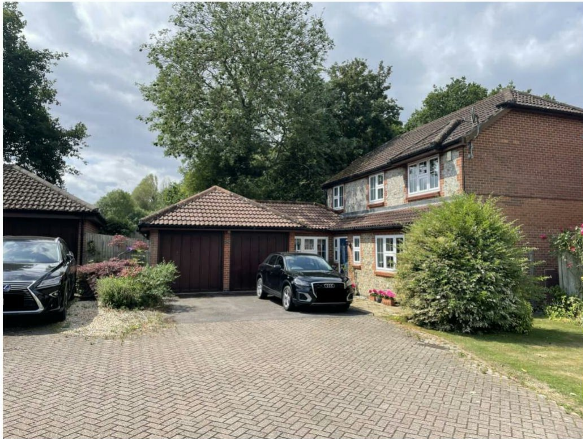
View of the front elevation,
