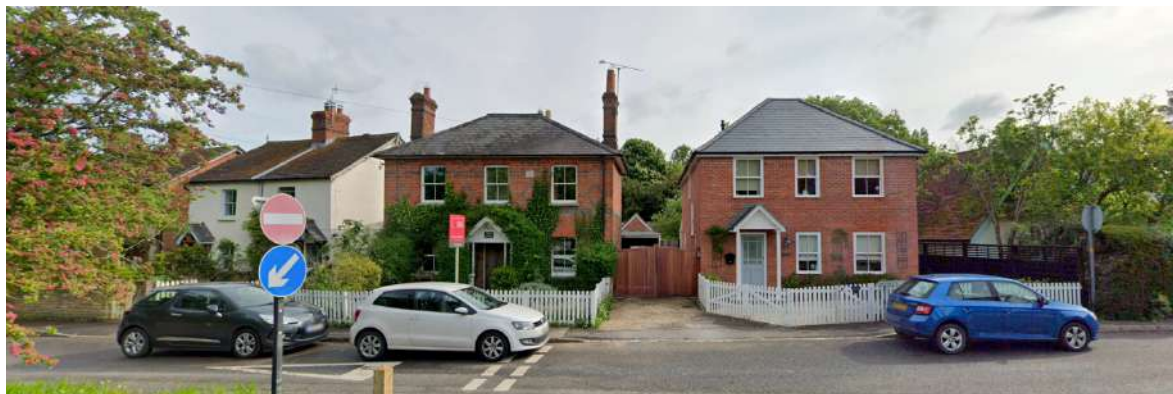
L to R – Rowan Cottage, Spring Cottage, and Bramble Cottage on Winkfield Row. Note, red brick, slate roof, projecting gable porch, 4 pane windows set beneath eaves and chimneys – details which influenced Plot 1 design.
