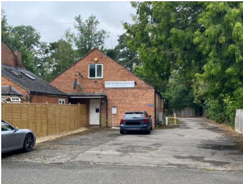
Front elevation of clubhouse. Note flank to flank tarmacadam.
