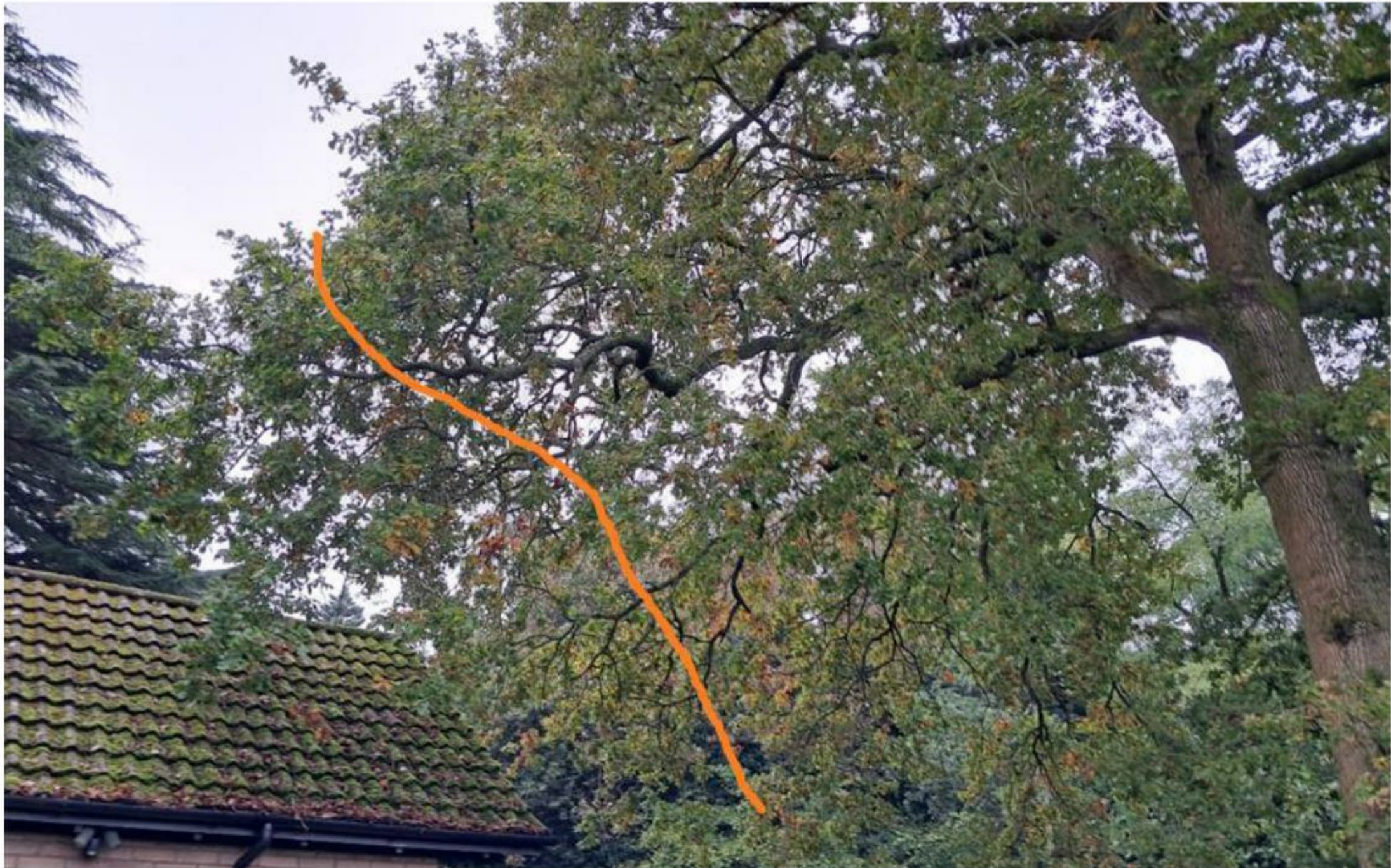
Photo 1 –Branches from tree touching roof of 18 Byron Drive
