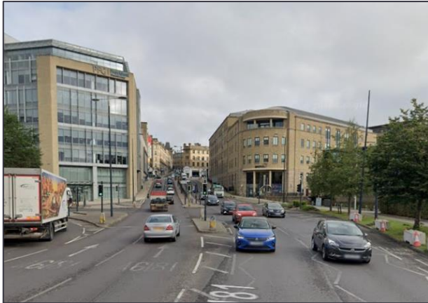
Signal Controlled Crossing – West of the Junction Mills Building
