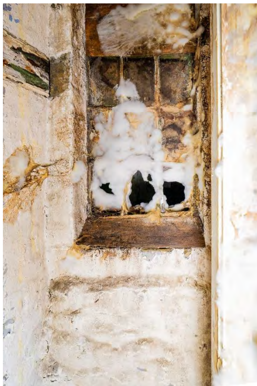
Photo 34: Detail of original window in basement, facing east
