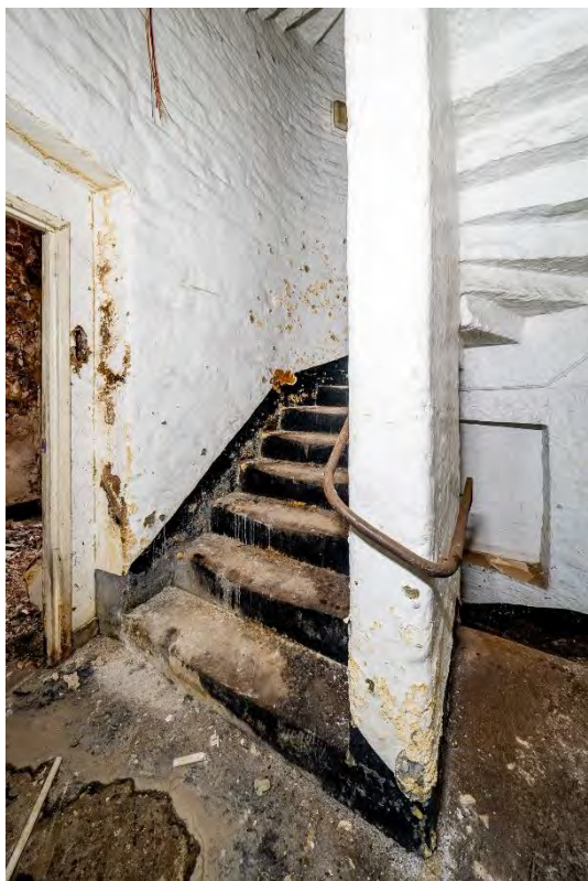
Photo 20: Winder stair (ground floor)
