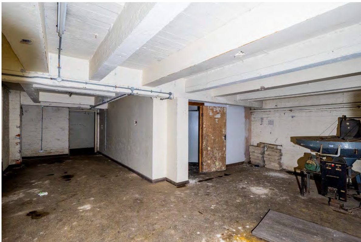
Photo 42: Central rooms of the north range basement, facing northwest
