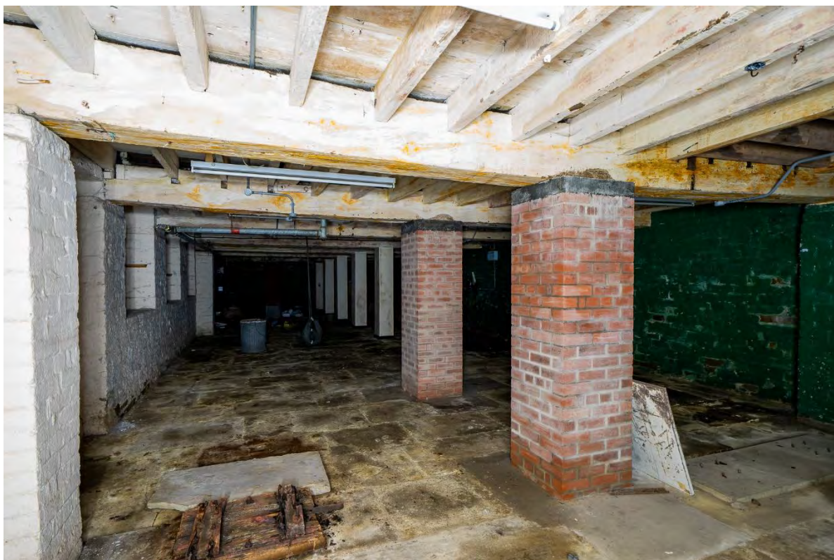
Photo 31: Overview of basement below the south range, facing east
