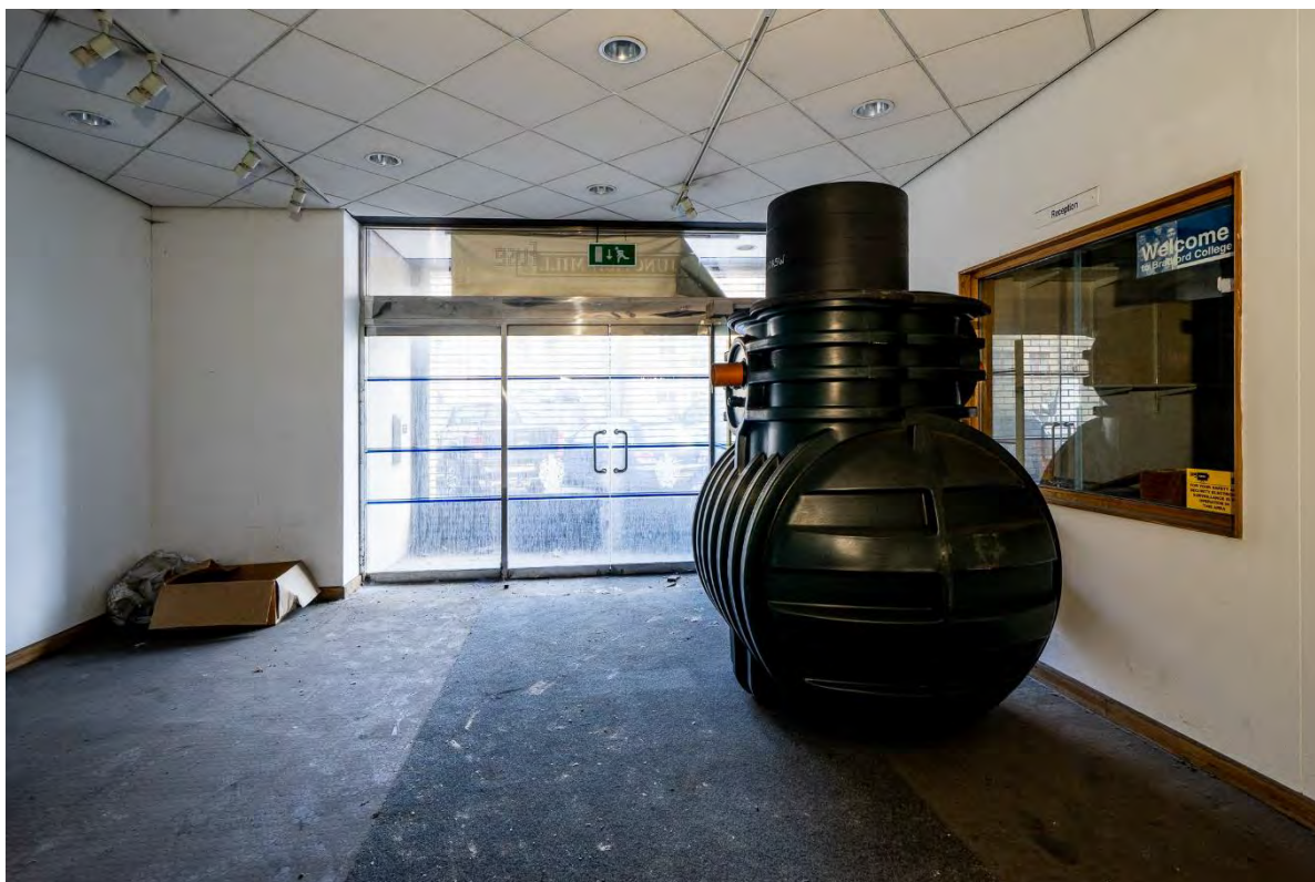
Photo 39: Modern lobby, facing north
