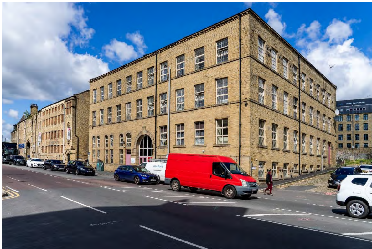
Photo 51: View northwest to Soho Mill and Holmefield Buildings from Westholme Street
