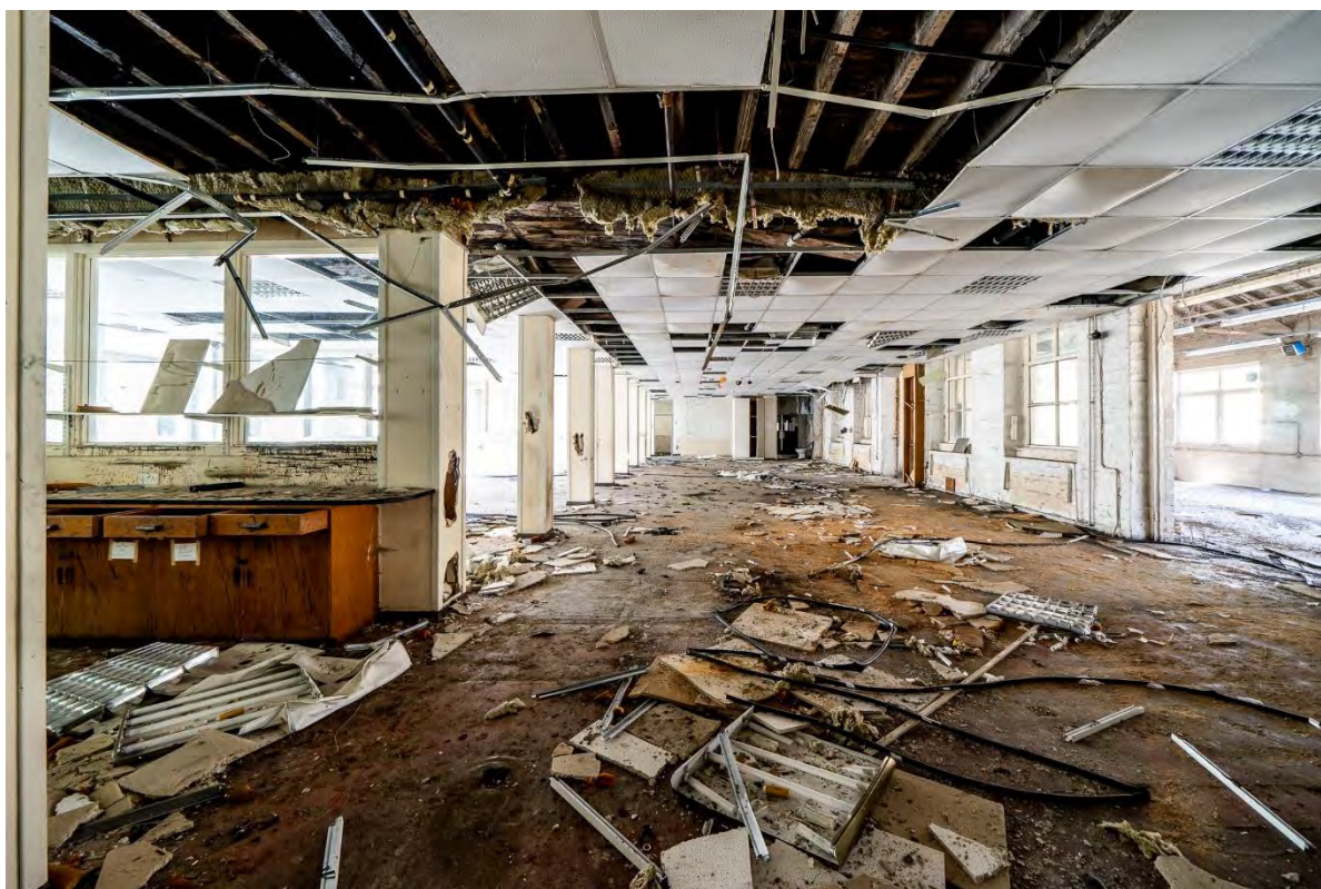
Photo 11: Second floor open-plan room of the south range, facing west
