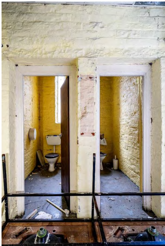
Photo 22: South range toilets (second floor)
