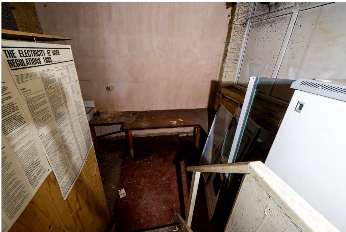
Photo 29: Interior of mezzanine room within the former engine house, facing south
