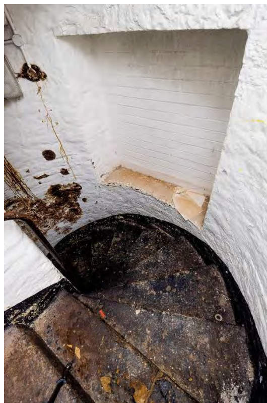
Photo 19: Winder stair, view down to basement
