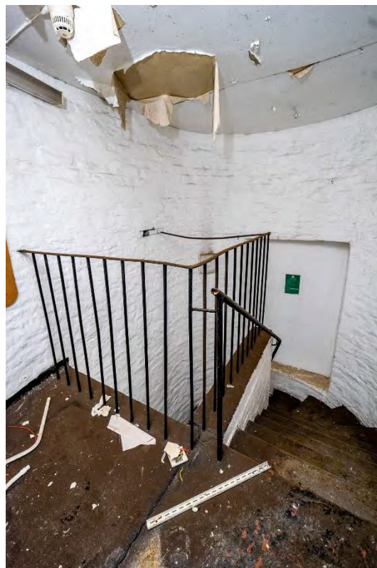
Photo 21: Winder stair (third floor)
