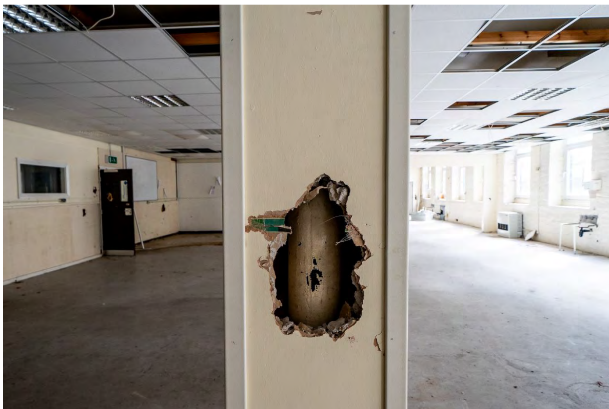
Photo 15: Boxed-in first floor column
