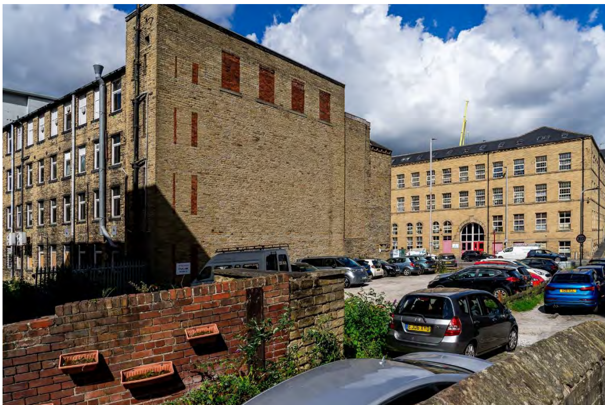
Photo 54: View northwest past the Site from Westholme Street towards Soho Mill
