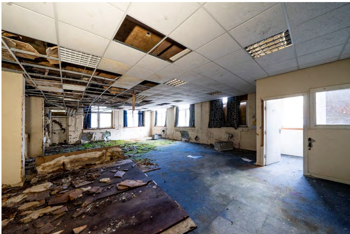
Photo 36: Western room of north range (ground floor)
