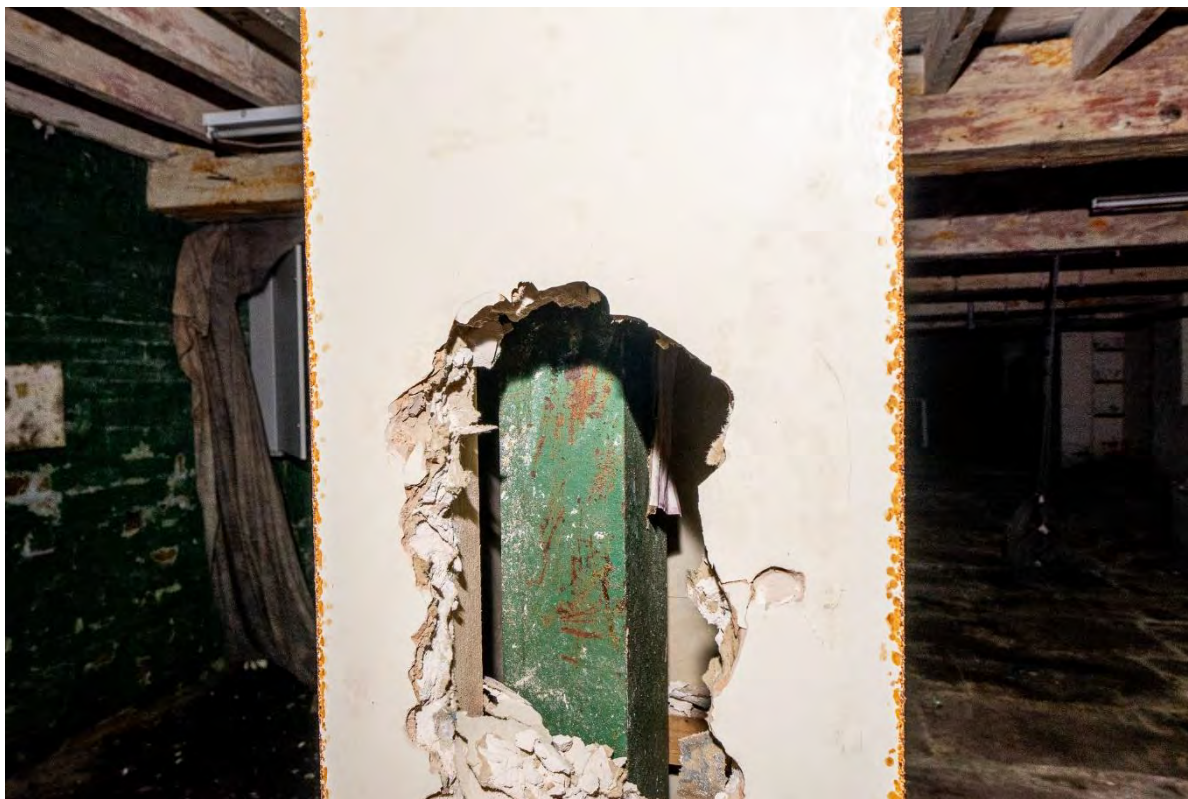
Photo 32: Column in basement
