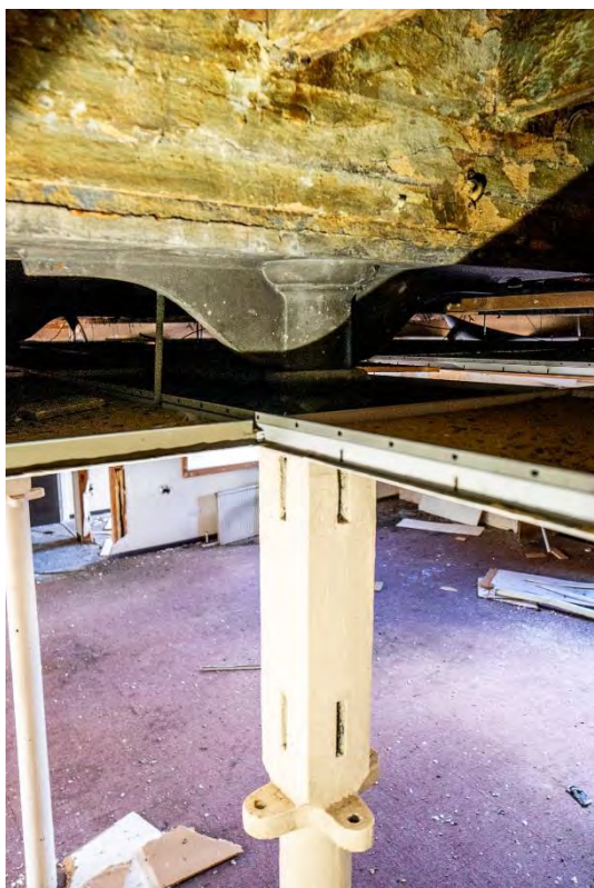
Photo 18: Exposed bracket to head of column (third floor)
