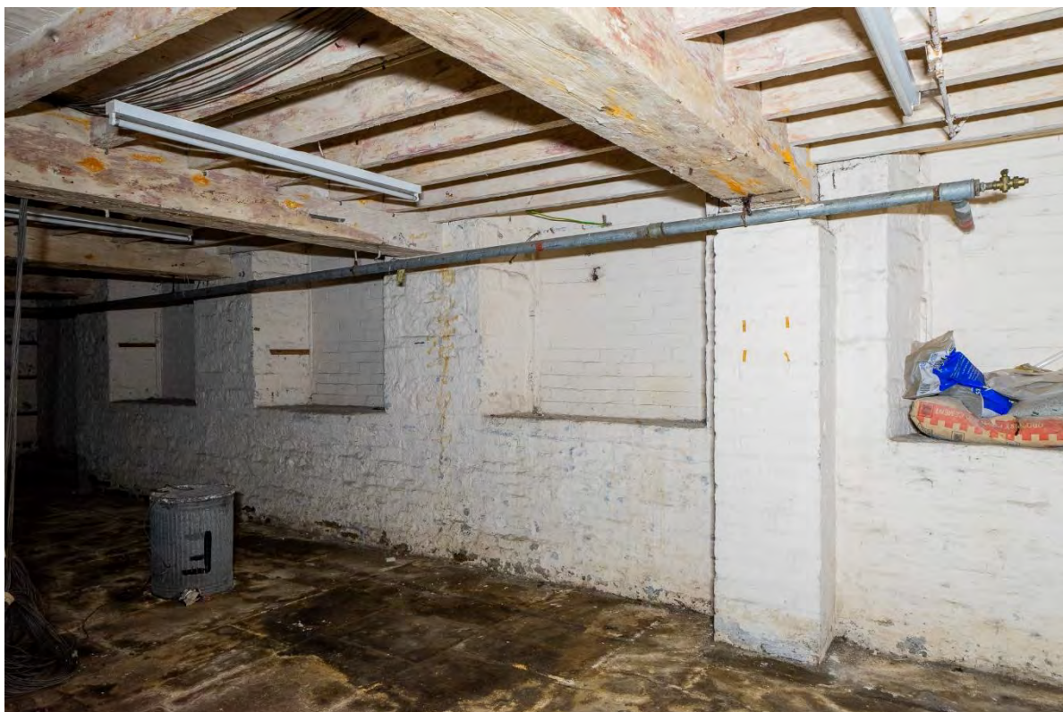
Photo 33: Window / lightwell openings within the basement, facing northwest
