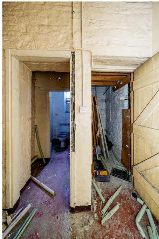
Photo 23: South range toilets (first floor)
