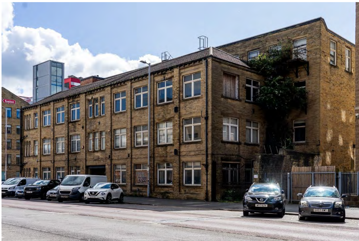
Photo 1: North and west elevations of Junction Mills
