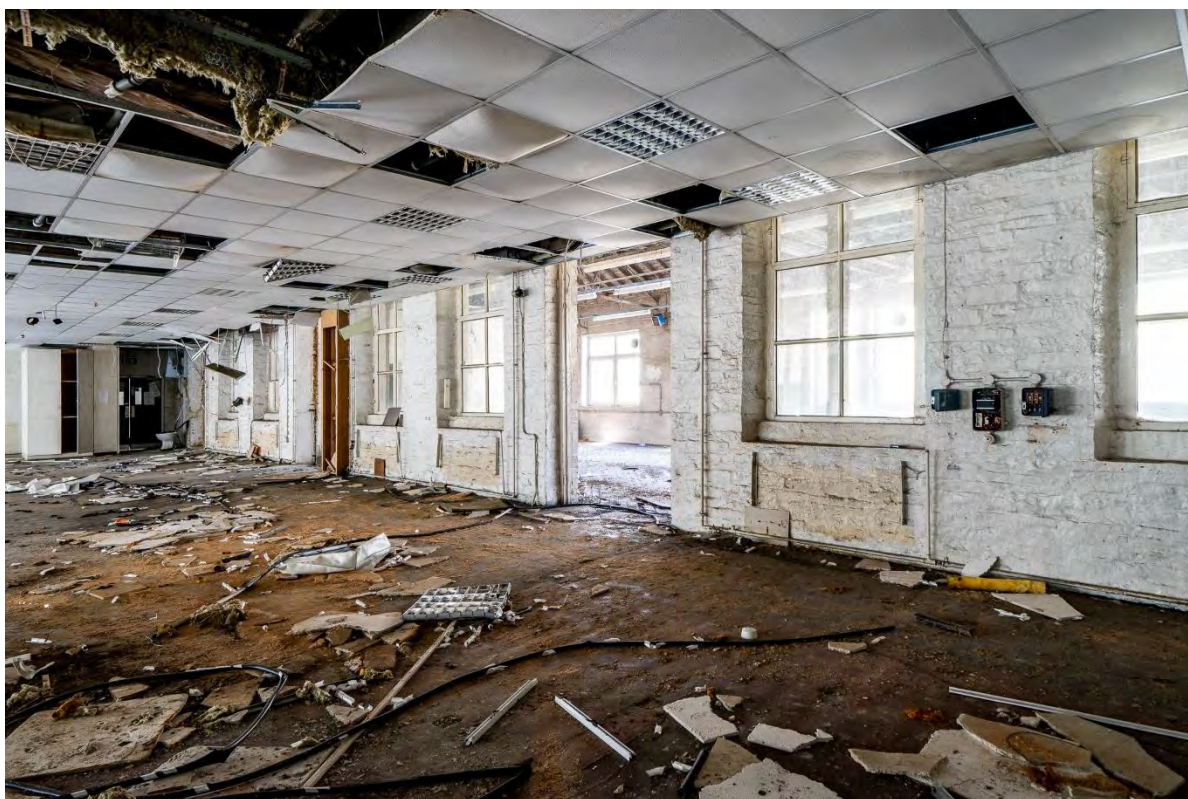
Photo 6: Windows to former north elevation of the south range, facing northwest (second floor)
