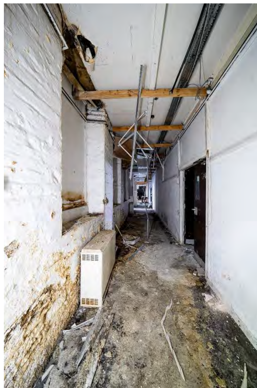
Photo 8: Ground floor corridor of the south range, facing east – note partitions
