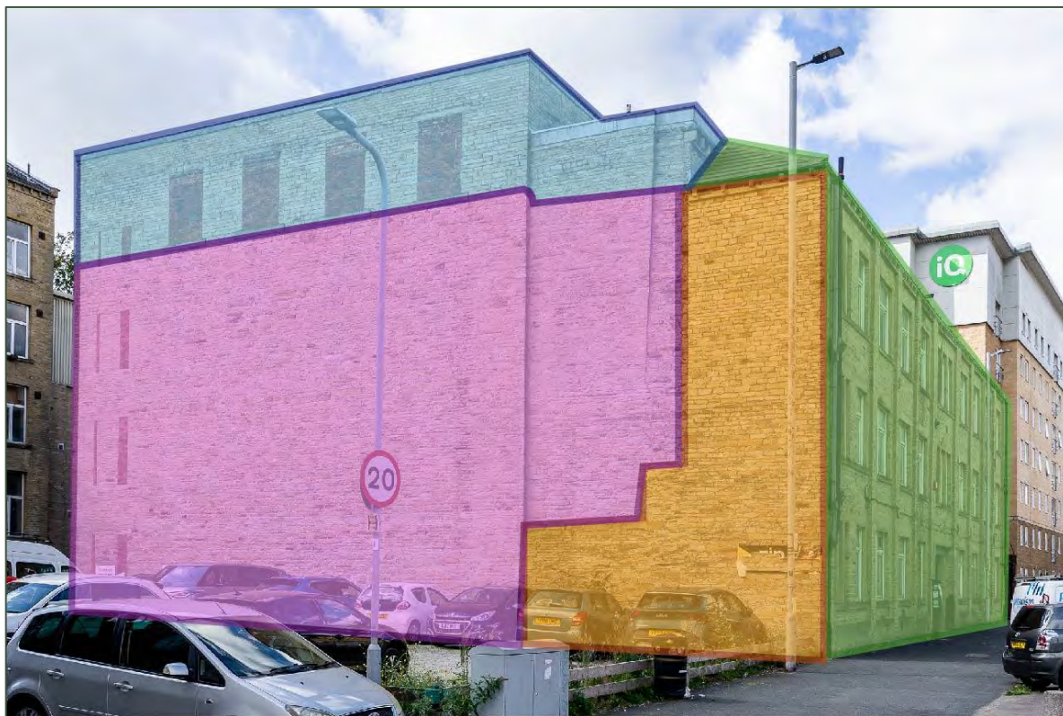
Plate 9: Phased elevations. Orange (Phase 1: 1852 – 1861), Pink (Phase 2: 1852 – 1861), Blue (possible Phase 3), Green (Phase 4: 1921 – 1934)
