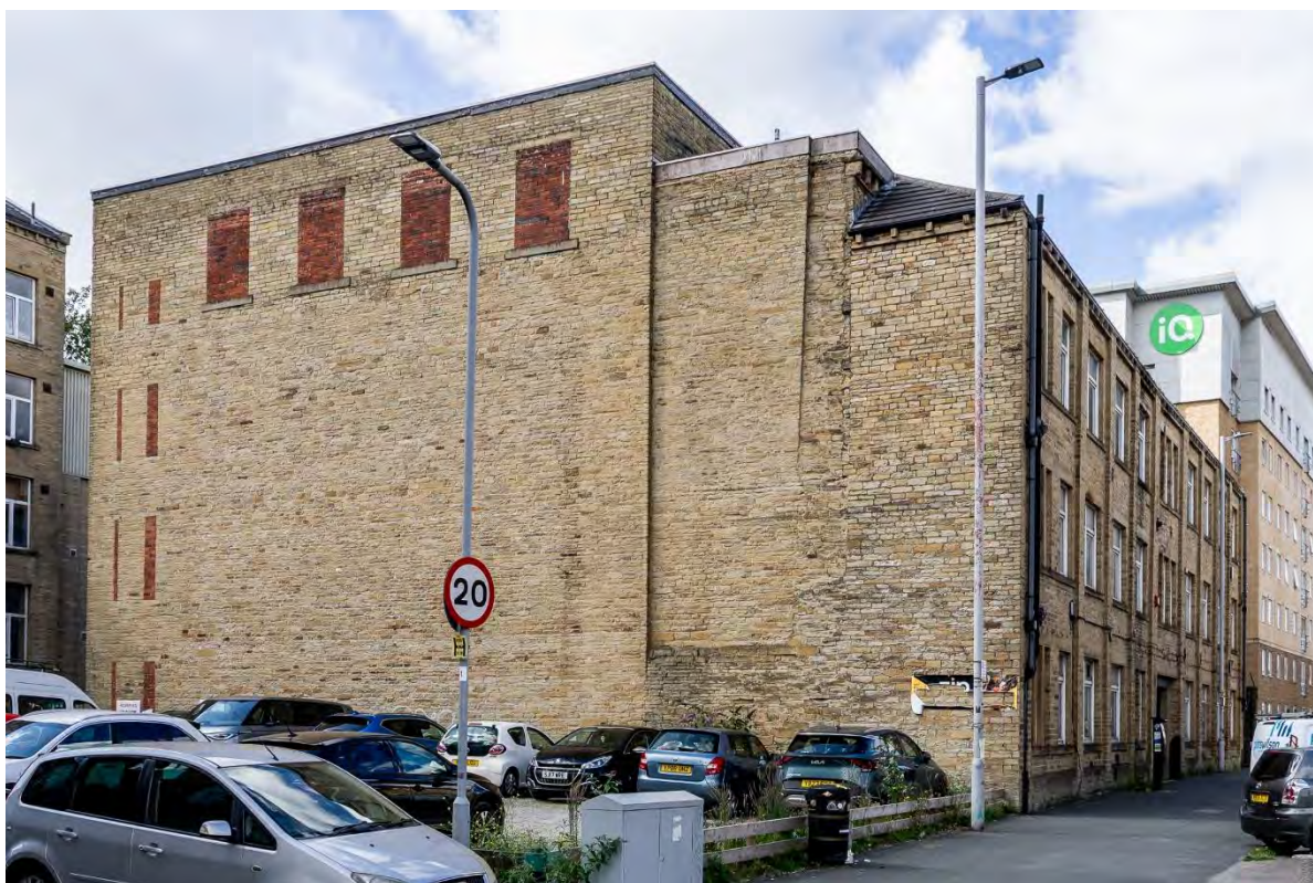
Photo 2: North and east elevations of Junction Mills
