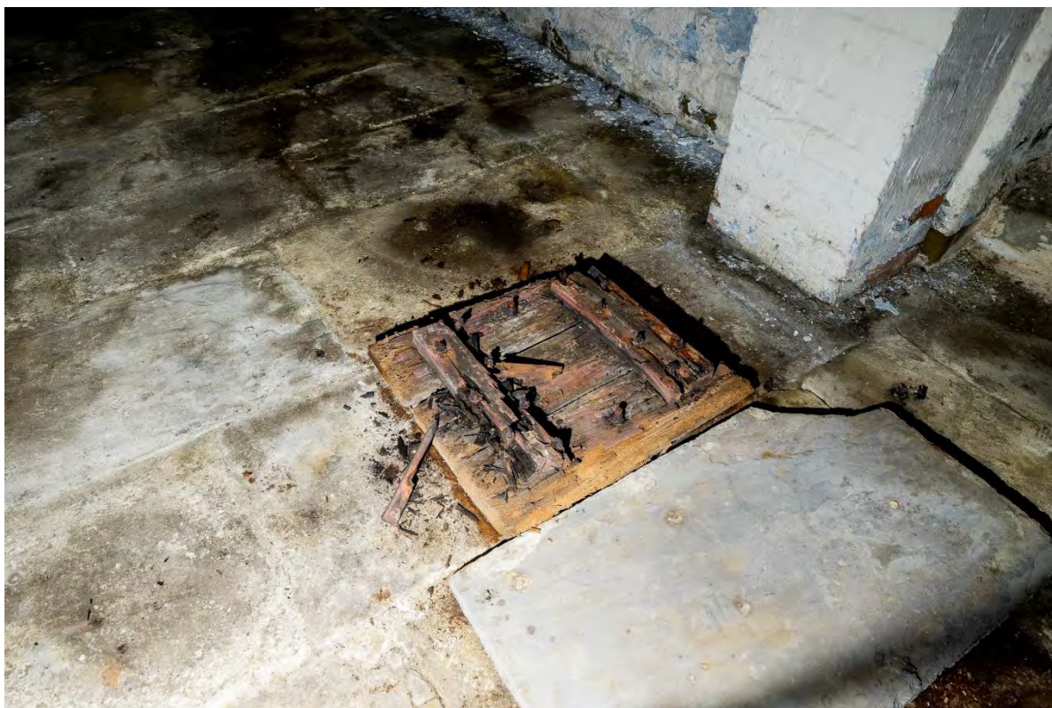
Photo 35: Possible plant base in basement
