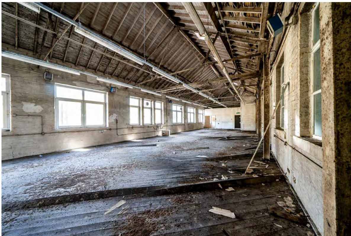
Photo 38: Open-plan second floor of the north range, facing east
