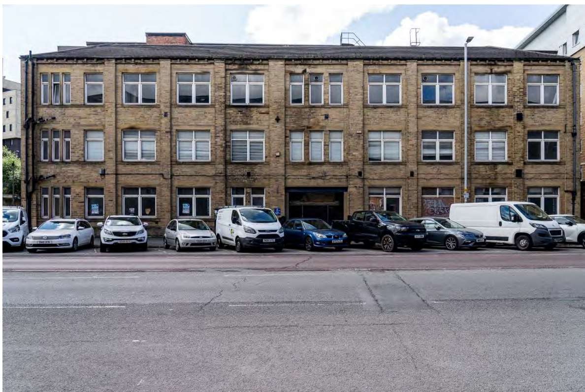
Photo 4: North and east elevations of Junction Mills
