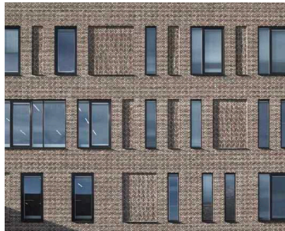
Materials (External) - Brickwork
