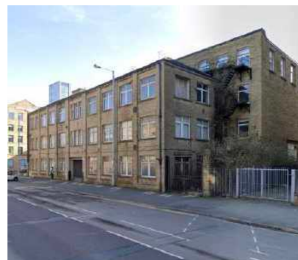
Existing Junction Mills building - To be demolished
