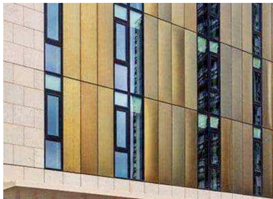
Materials (External) - Cladding
