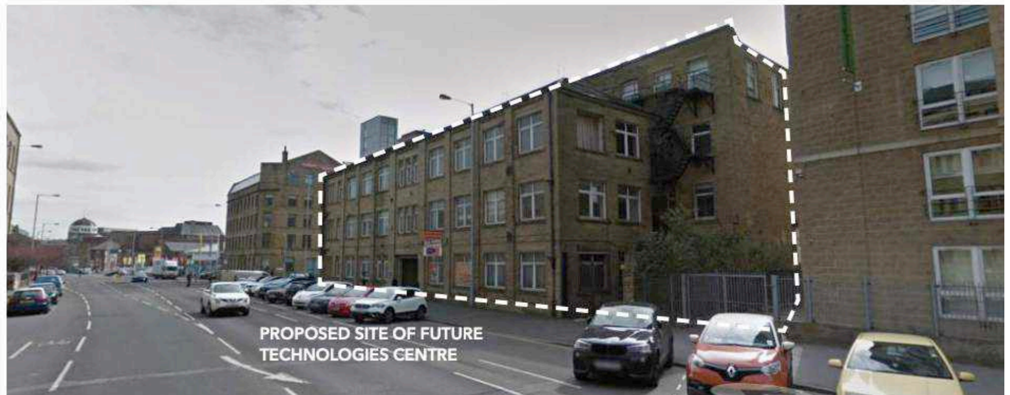
Junction Mills photos as existing
