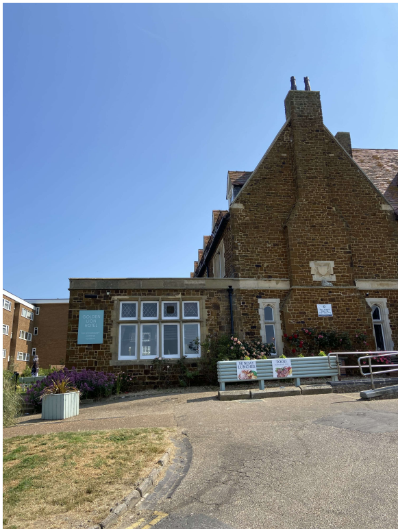
The south west corner extension.
