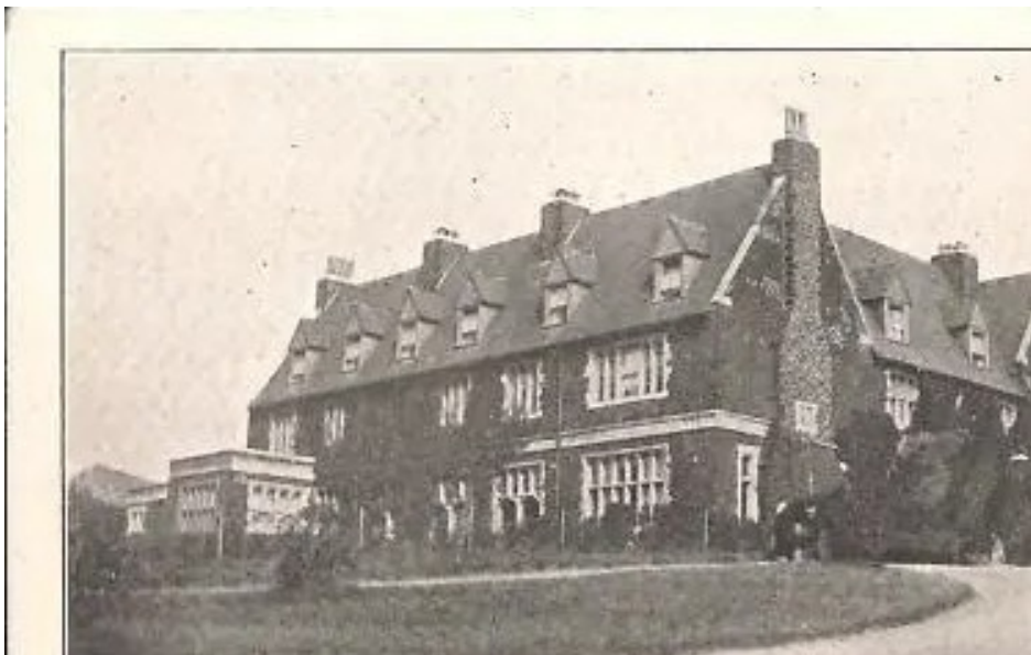
Photo showing the first extension only.
