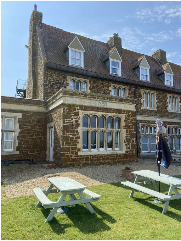
North West corner extension
