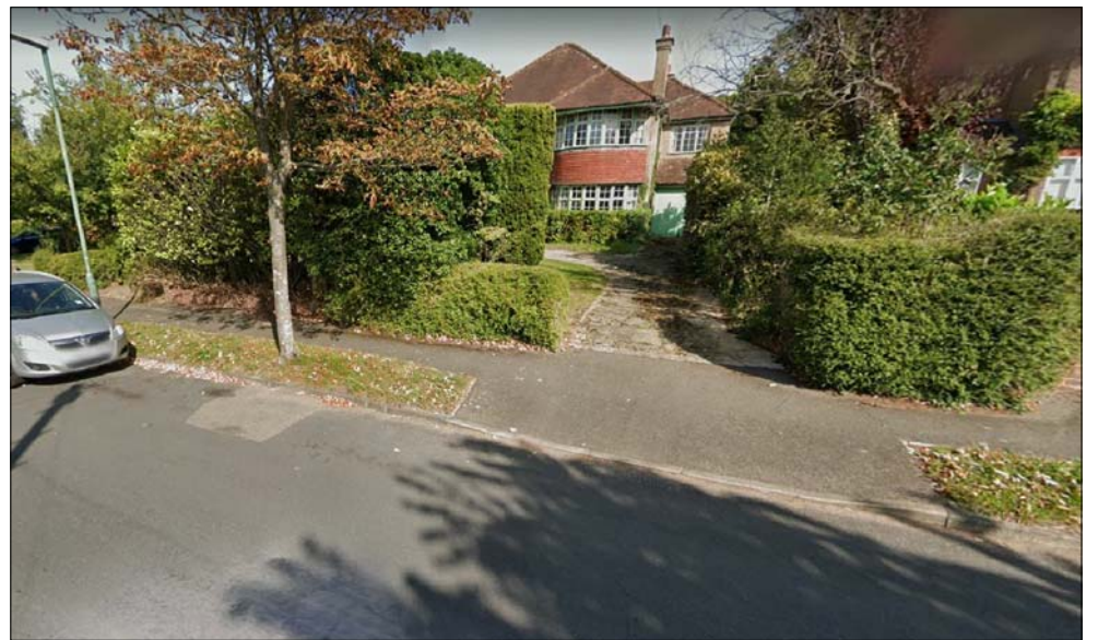
EXTERNAL VIEW OF No 52 HIGHER DRIVE ALLOWING DIRECT FIRE BRIGADE ACCESS AND SAFE ASSEMBLY POINT
