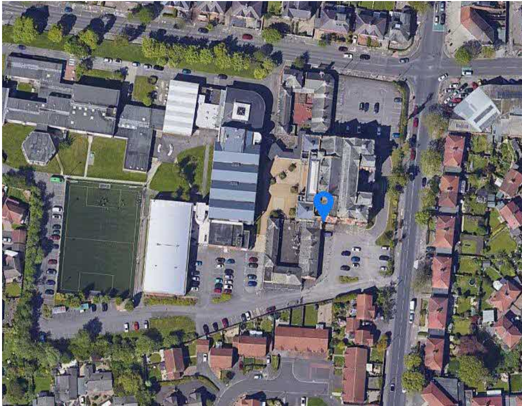
Figure 1 - An image illustrating the proposed location for the telecoms installation.
