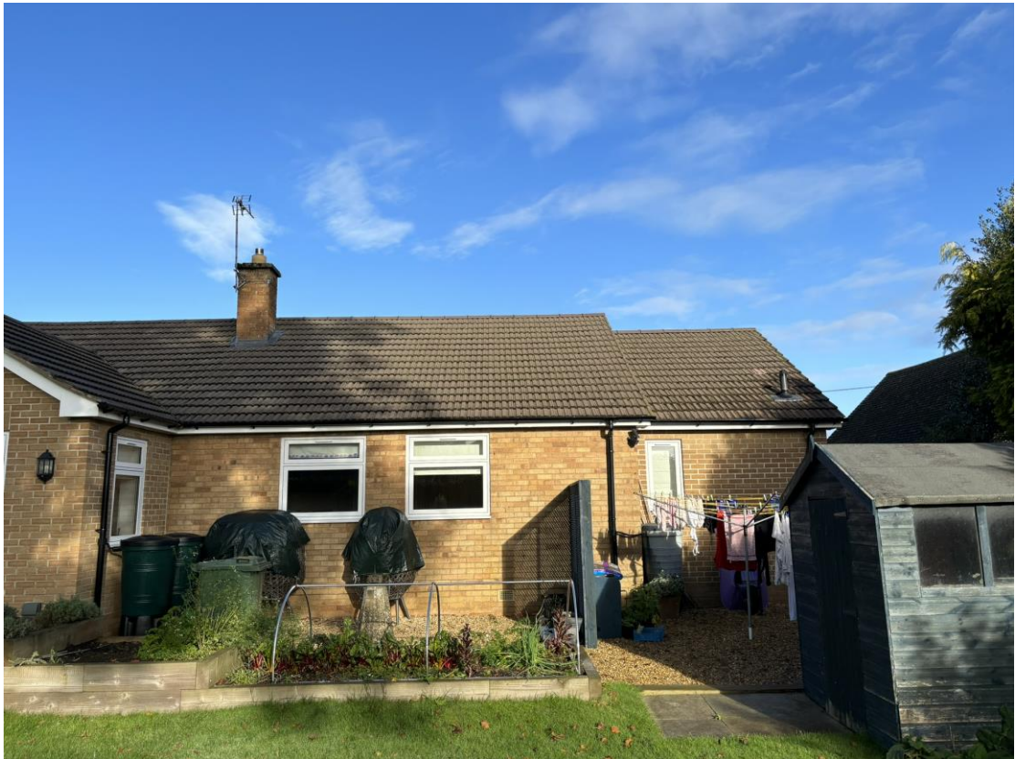
Above photo (top) – existing front elevation. Above photo (bottom) – portion of existing rear elevation.
