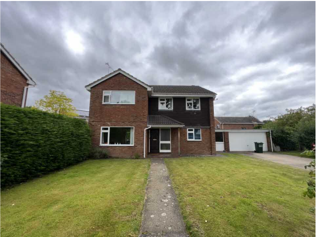
Photo 02. Front garden and elevation.
