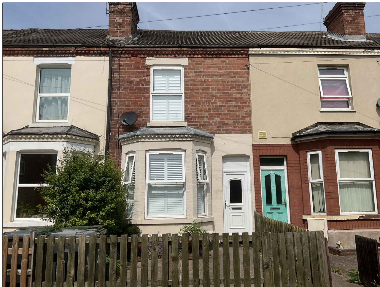
Application house No. 43 is in the middle. NB: Home to right has already had external wall insulation applied.
