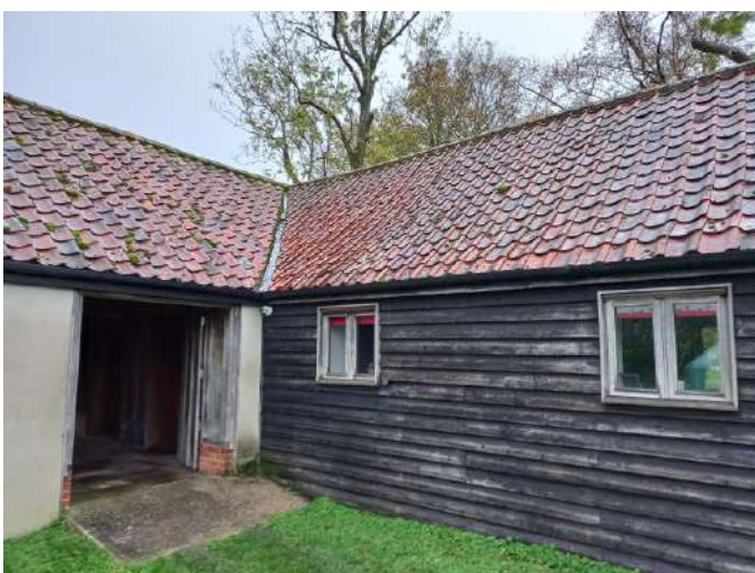
Figure 6: View of the northern site entrance.
