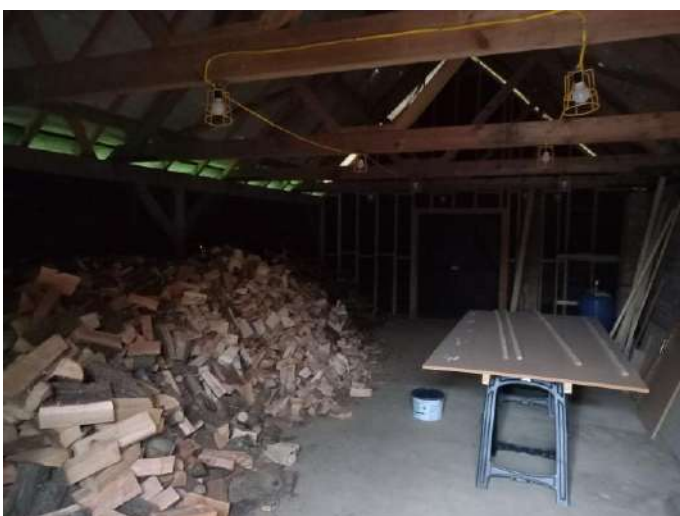
Figure 3: View inside one of the barns.
