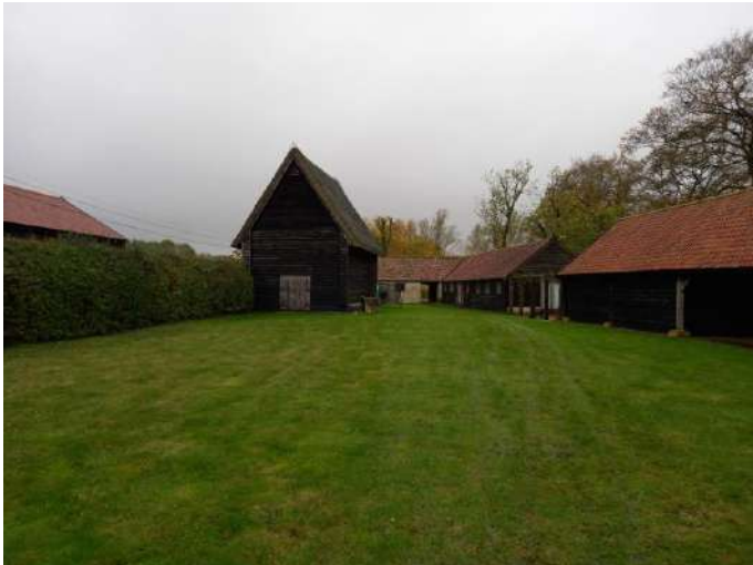
Figure 4: View of the site looking north-west.
