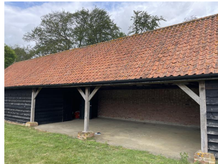
Fig.10 covered entrance area
