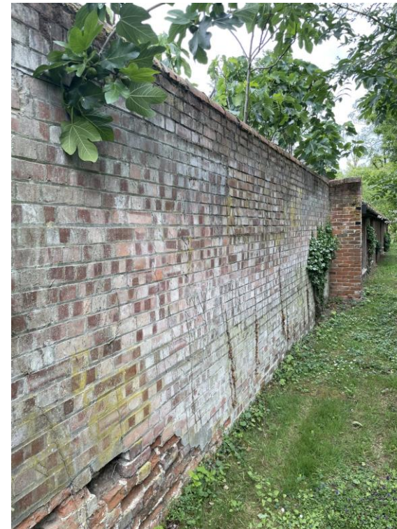
Fig.8 brickwork condition to elevation facing moat
