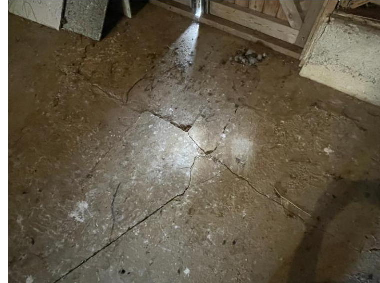
Fig.27 slab cracking
