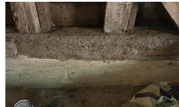
Fig.25 soleplate section with significant insect damage
