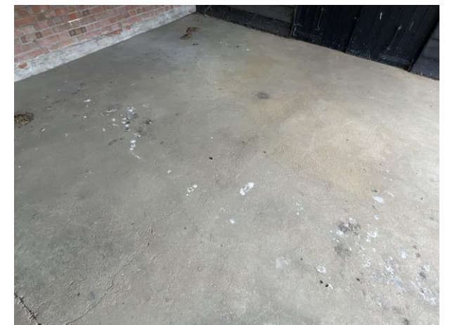
Fig.14 general view - concrete floor slab
