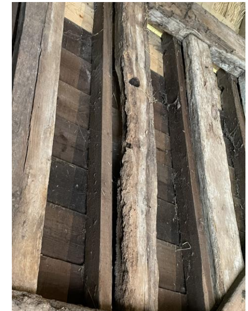
Fig.19 supplementary cladding supports
