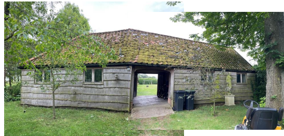
Fig.4 timber clad elevation to north-west
