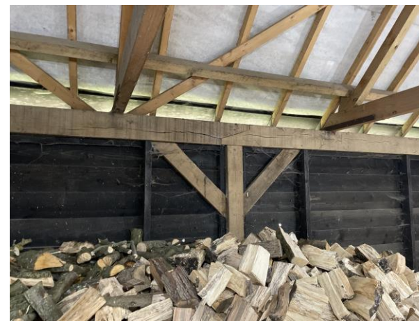
Fig.13 general view - visible timber frame
