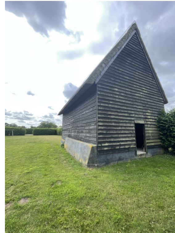
Fig.15 general external view
