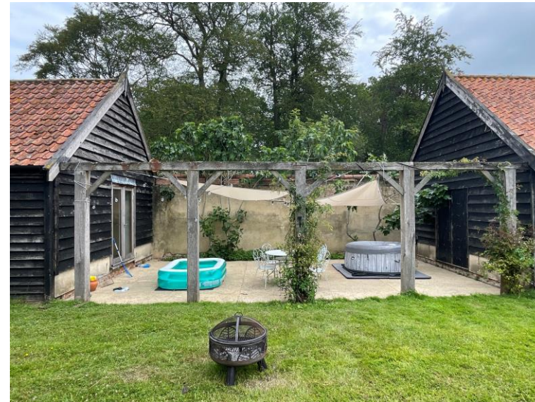
Fig.6 exposed timber frame
