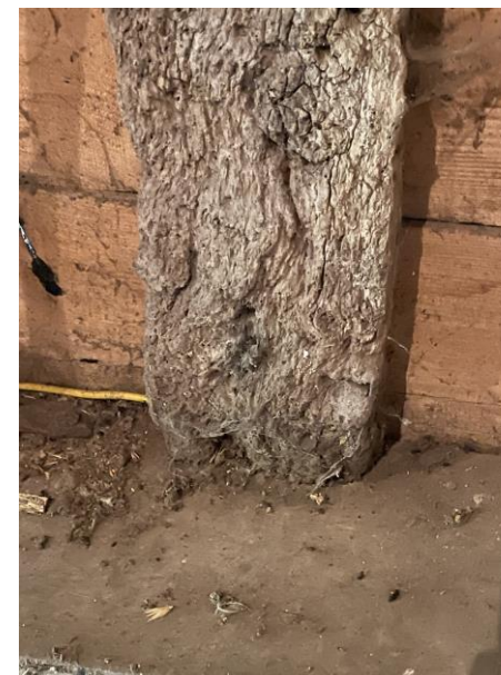
Fig.20 insect damage
