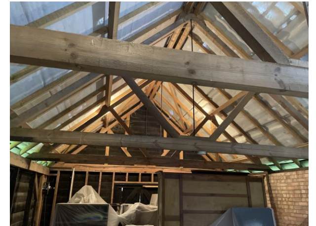
Fig.12 general view - internal roof condition
