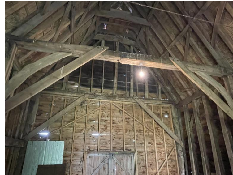
Fig.16 general internal frame view
