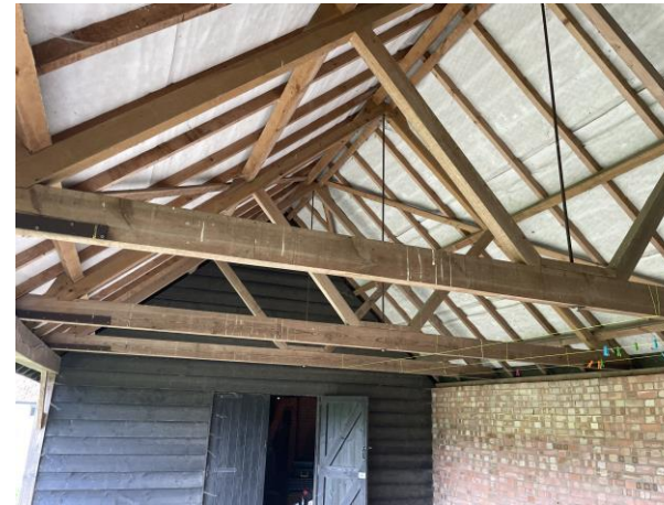
Fig.11 general view - roof condition over covered external area
