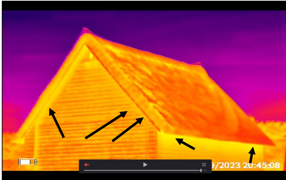
Figure 5: Locations of bat emergences during surveys on B1 shown by black arrows on thermal camera image.
