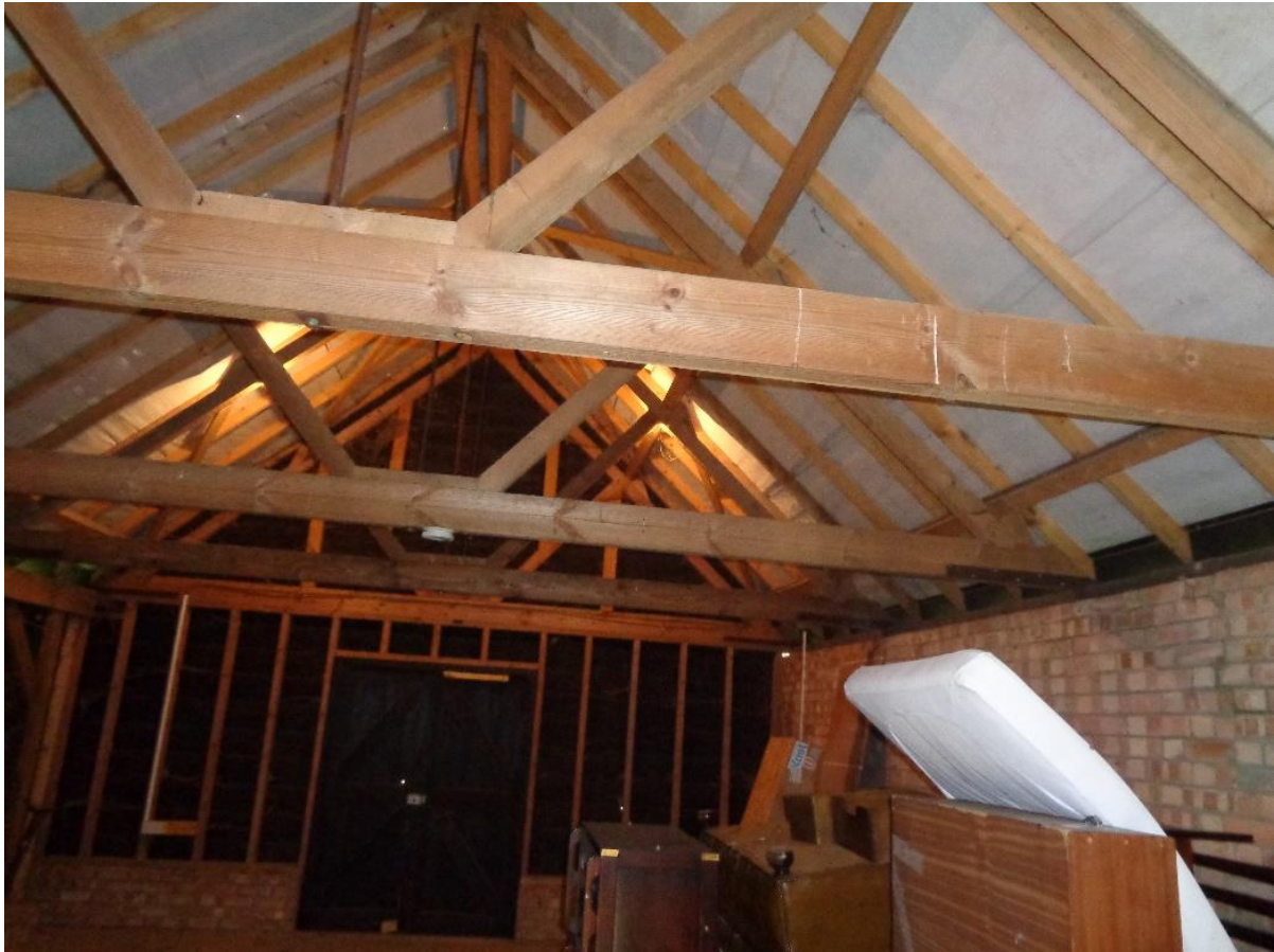
Interior of Building B
