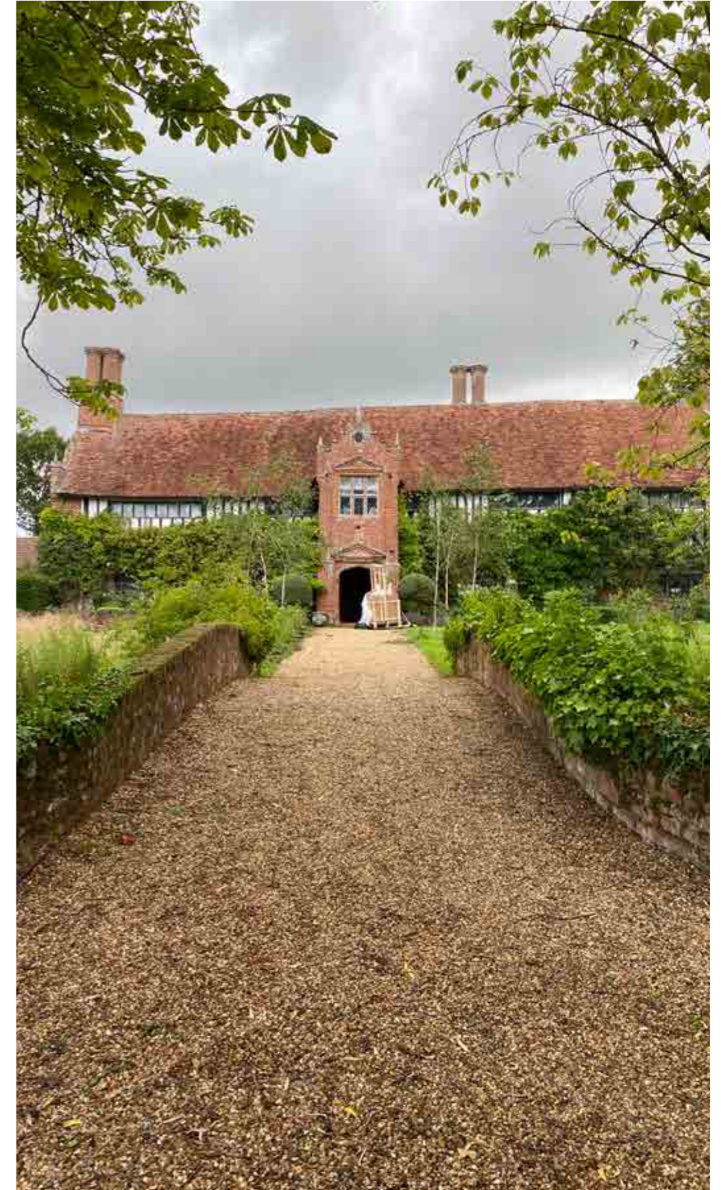
Fleming Hall Entrance Path
