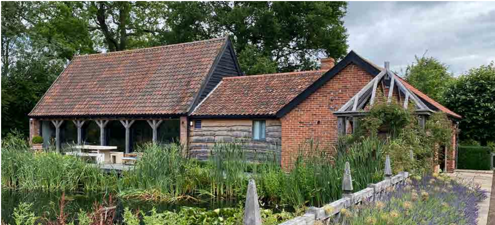
Garden room with glazed opening overlooking the pond. Design and Access Statement
