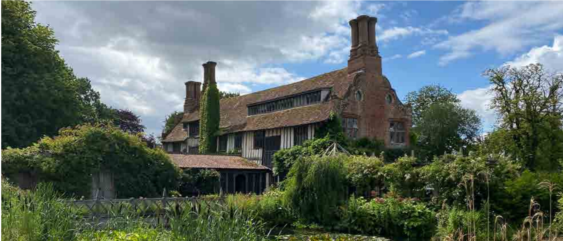
View towards Fleming Hall over moat
