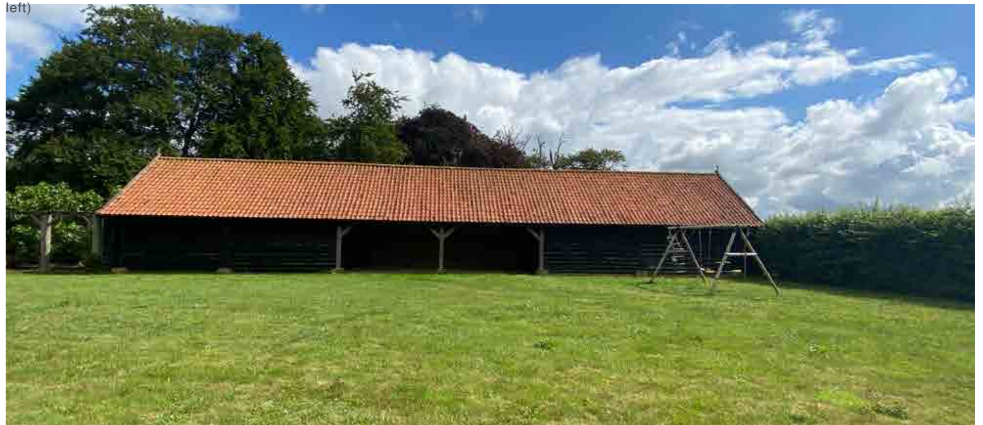
Outbuilding within site
