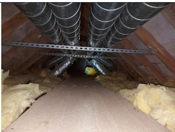
Photograph 11. B2 loft area with crawl space.
