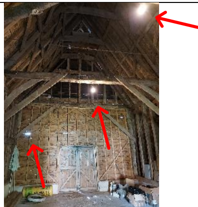
Photograph 6. East elevation internally showing access points.
