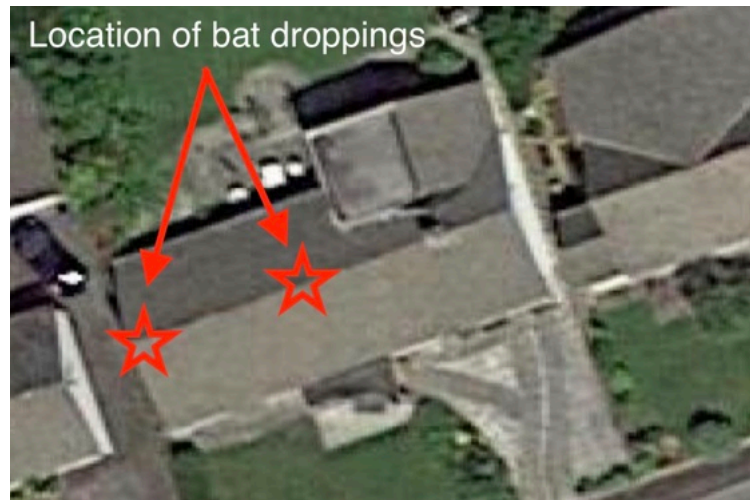
Plate 10. Location of areas of localised bat droppings
