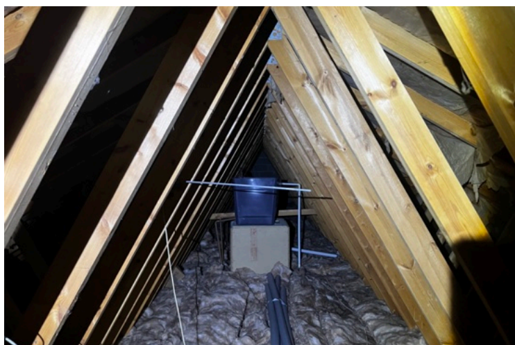
Plate 6. Internal view of attic
