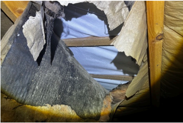
Plate 7. Multiple liners beneath roof tiles
