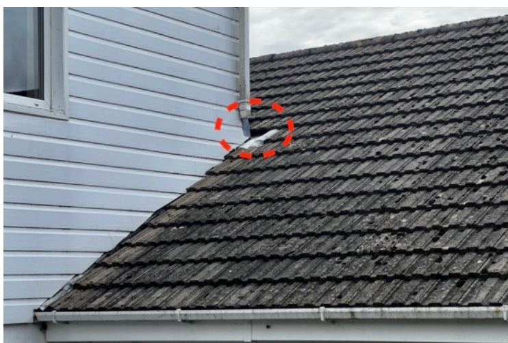
Plate 4. Gaps to tiles close to extension
