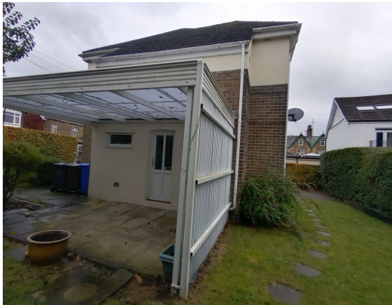
Side view showing veranda area and existing brick-built side extension
