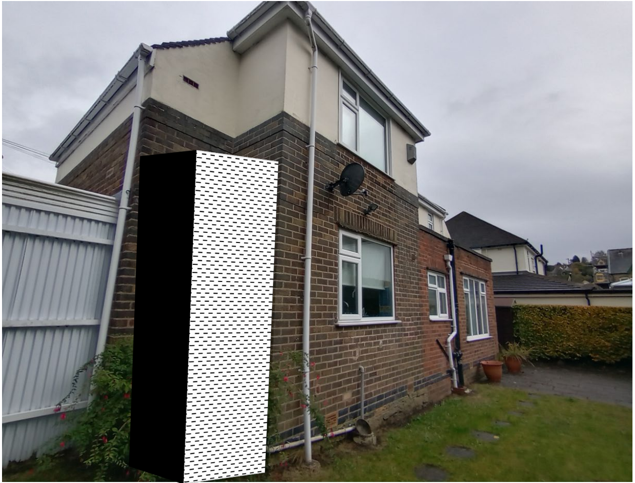
Rear/side view with an illustration of the proposed in-fill rear 'single storey' extension (height to match existing single storey extension to right) – exterior walls to be rendered in soft white – with wood composite cladding applied to exterior of garage section + existing side extension + proposed rear in-fill extension.
