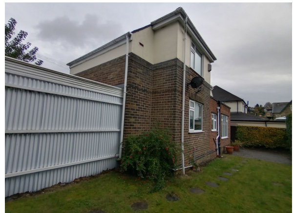
Rear/side view showing existing void space for proposed In-fill rear extension
