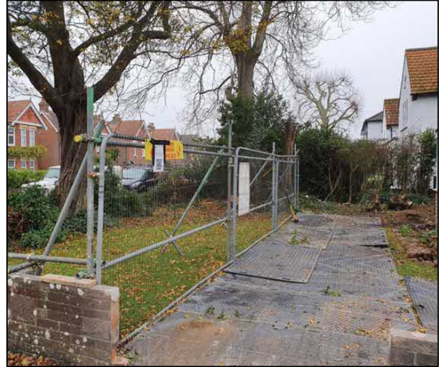
GP2: Tree protection barriers & trackmat ground protection
