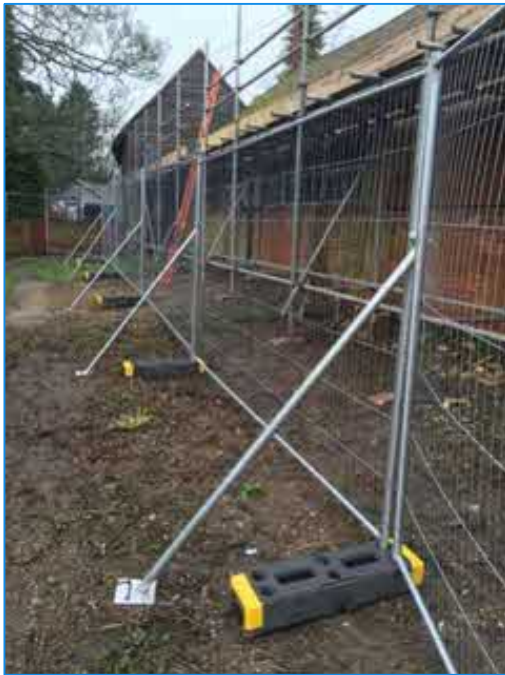
TPF 3: Alternative fencing option: orange boots with backstay
