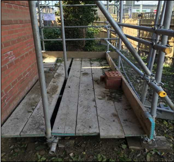
GP1: Tree protection barriers and scaffold ground protection
