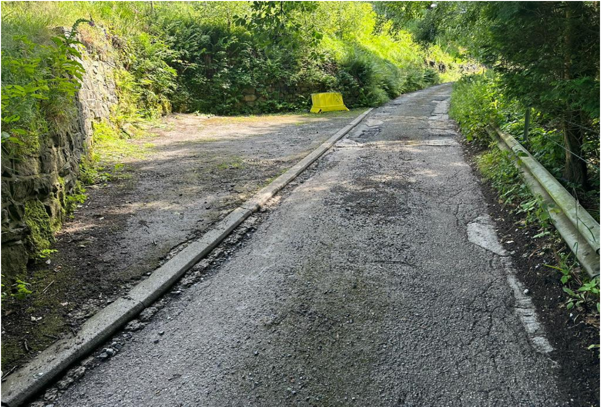
7. Hard standing above corner
