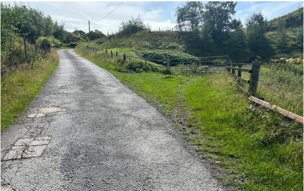
8. Layby bottom of quarry
