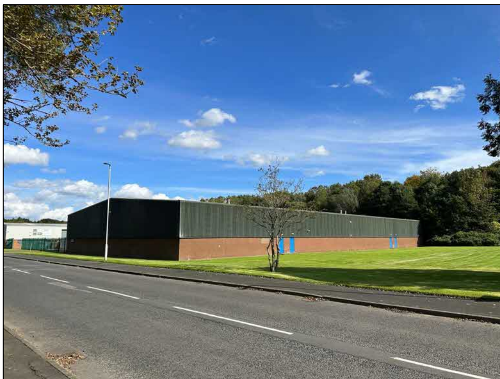
Figure 9 The only building on site, a large industrial unit with negligible potential for bat roosting
