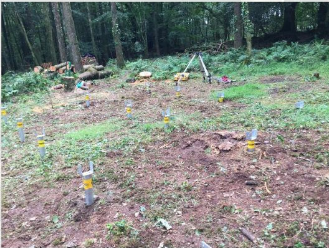
Screws installed ready for base frame
