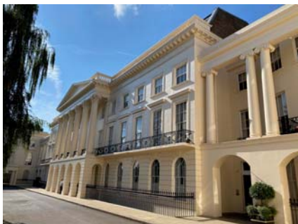
Frontage (N.E.) facing Regents Park.
