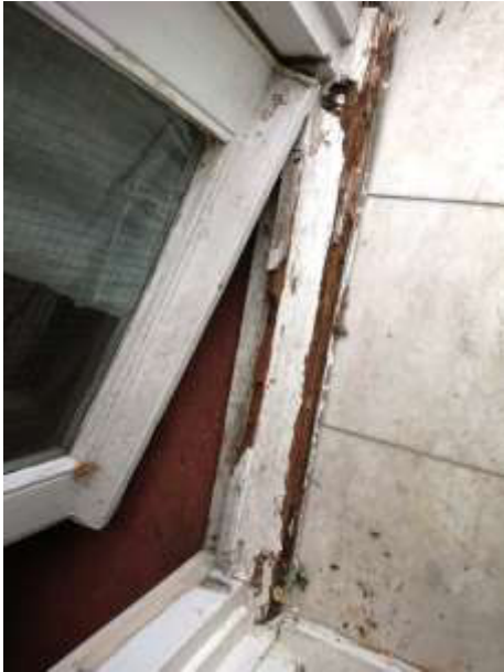
ROTTED DOOR THRESHOLD
