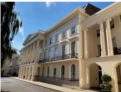
Frontage (N.E.) facing Regents Park.
