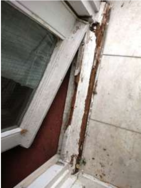
ROTTED DOOR THRESHOLD
