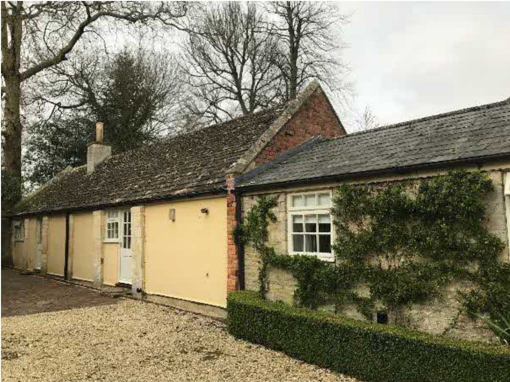
Photograph 10. The south aspect of the Stable Cottage. The area beneath the slate-tiled section contains a roof space. The stone tiles have occasional gaps beneath.
