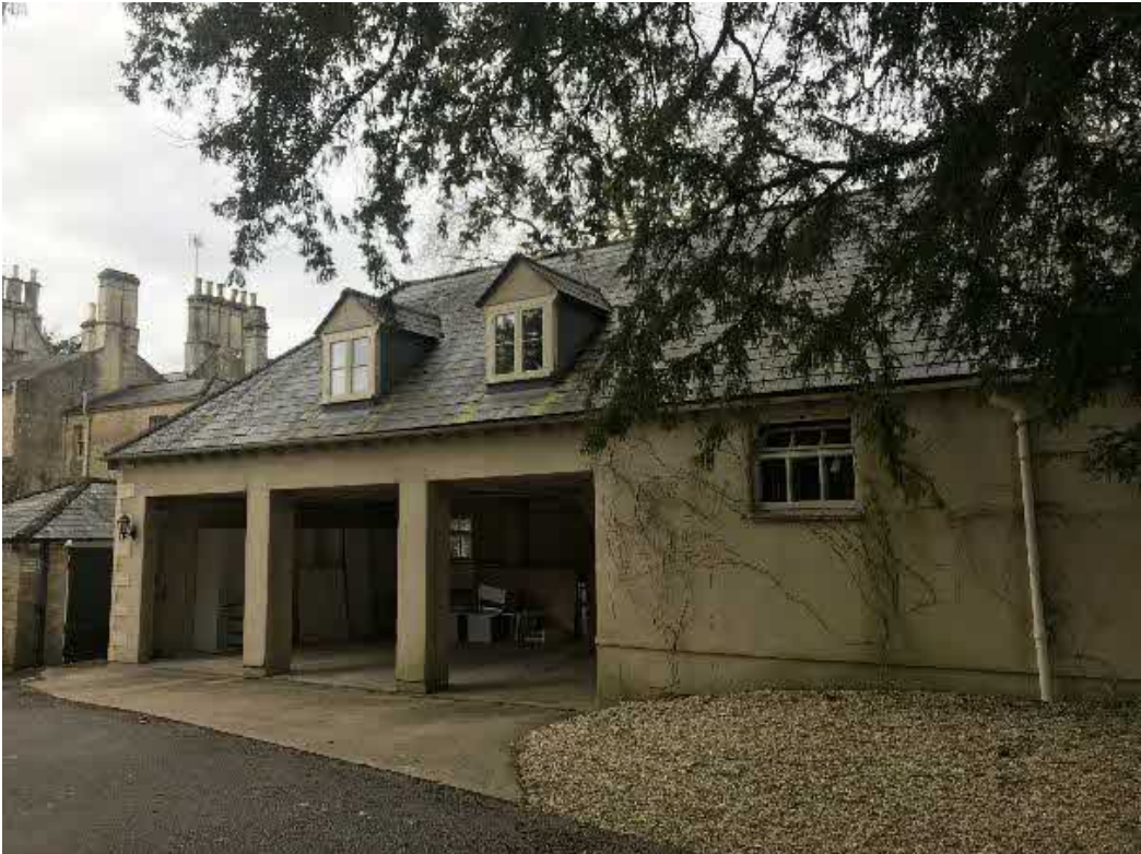
Photograph 10. The south aspect of the Stable Cottage. The area beneath the slate-tiled section contains a roof space. The stone tiles have occasional gaps beneath.
