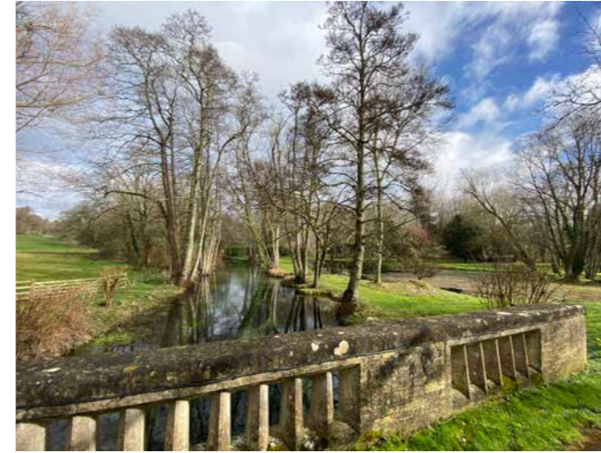
Fig.03. Ampney Brook - Bridge
