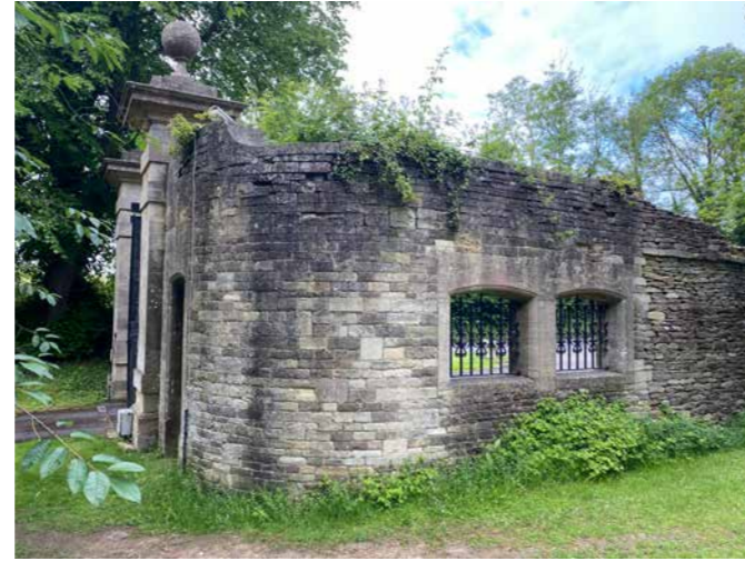
Fig.02. Entrance Gate - Side
