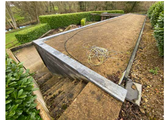
Fig.08. Grounds Building - Building roof
