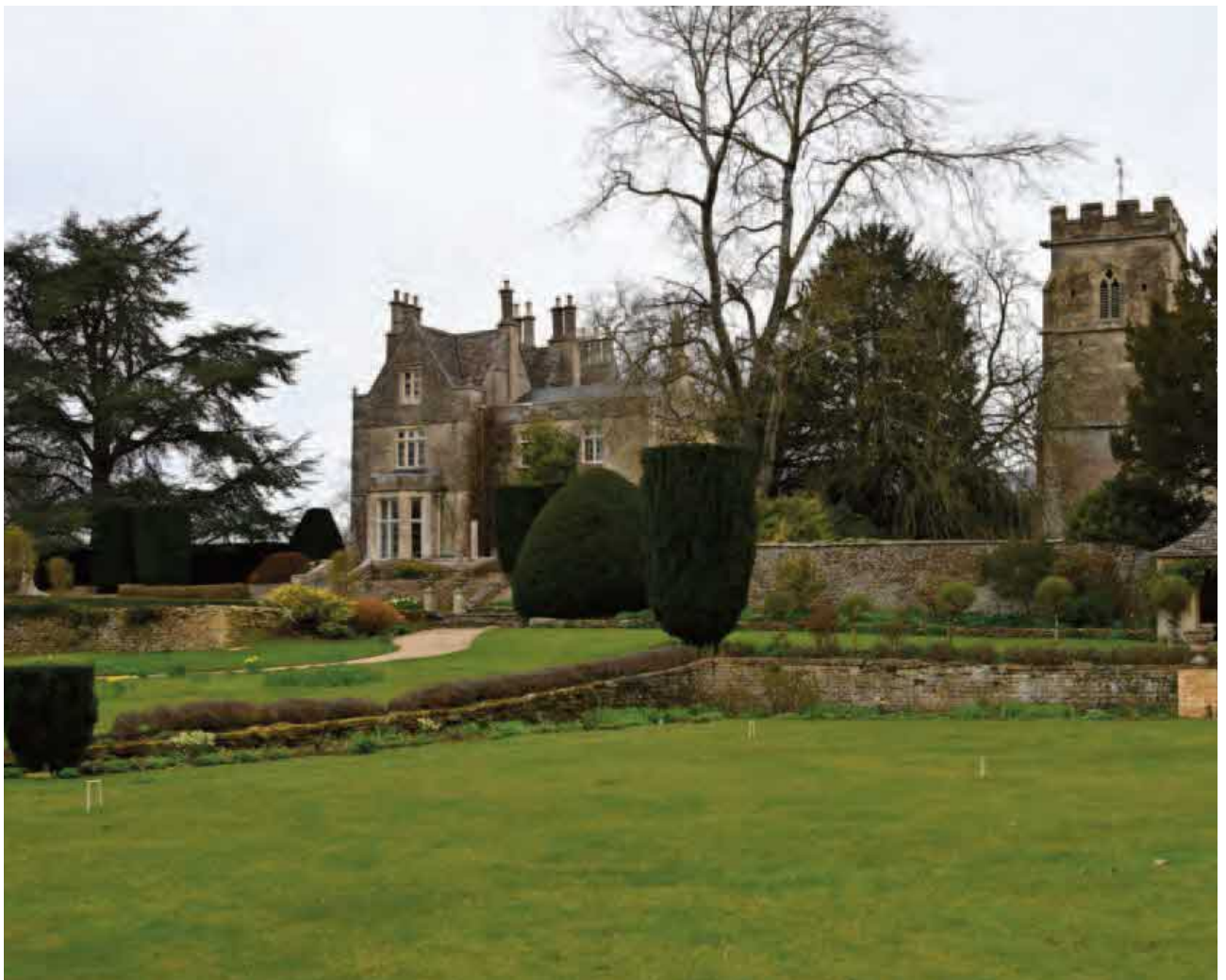
Fig 1. The current house, seen in its carefully landscaped grounds immediately adjacent to the parish church which dates back to Saxon times.
