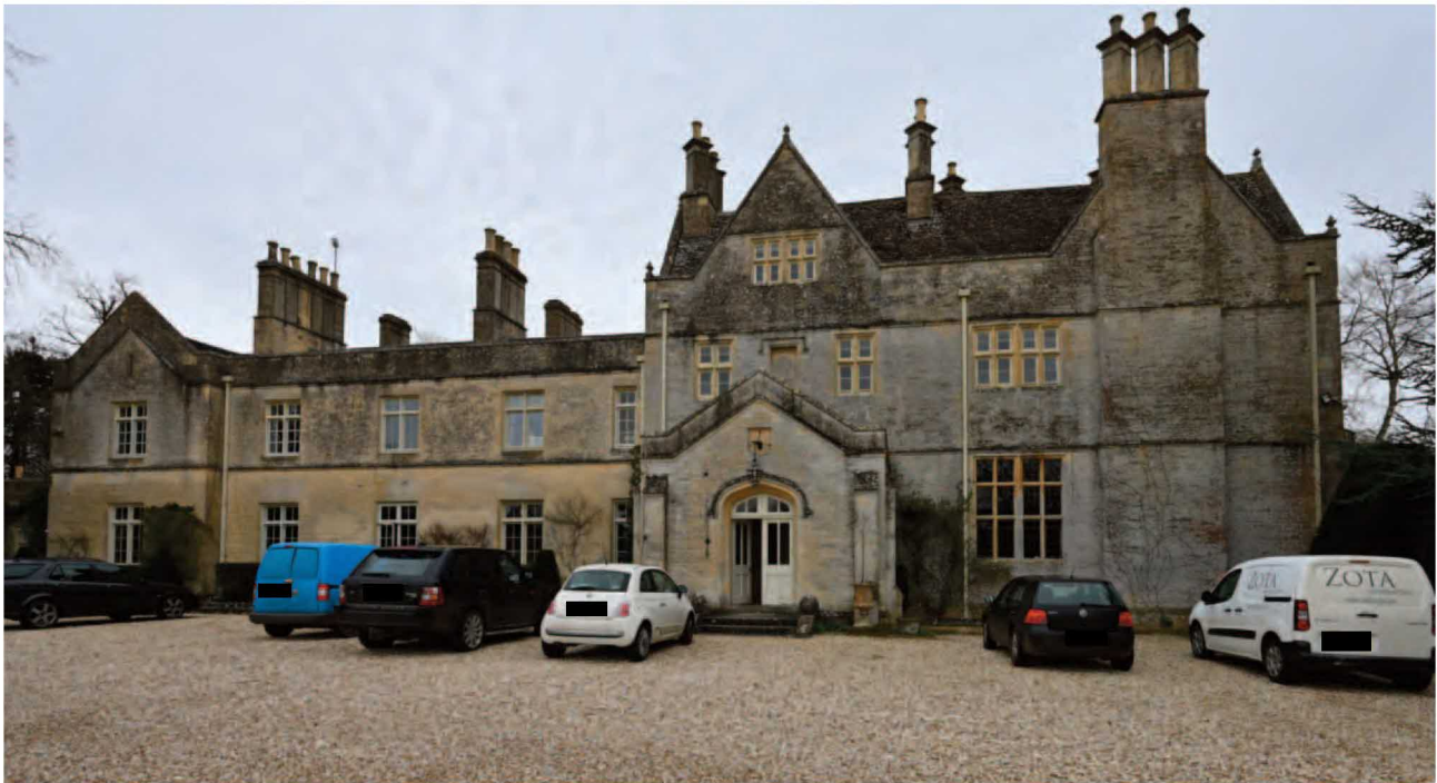
Fig 5. The taller 17th century principal range on the right with the early 19th century double pile north range on the left terminating in a short later 19th century cross wing.
