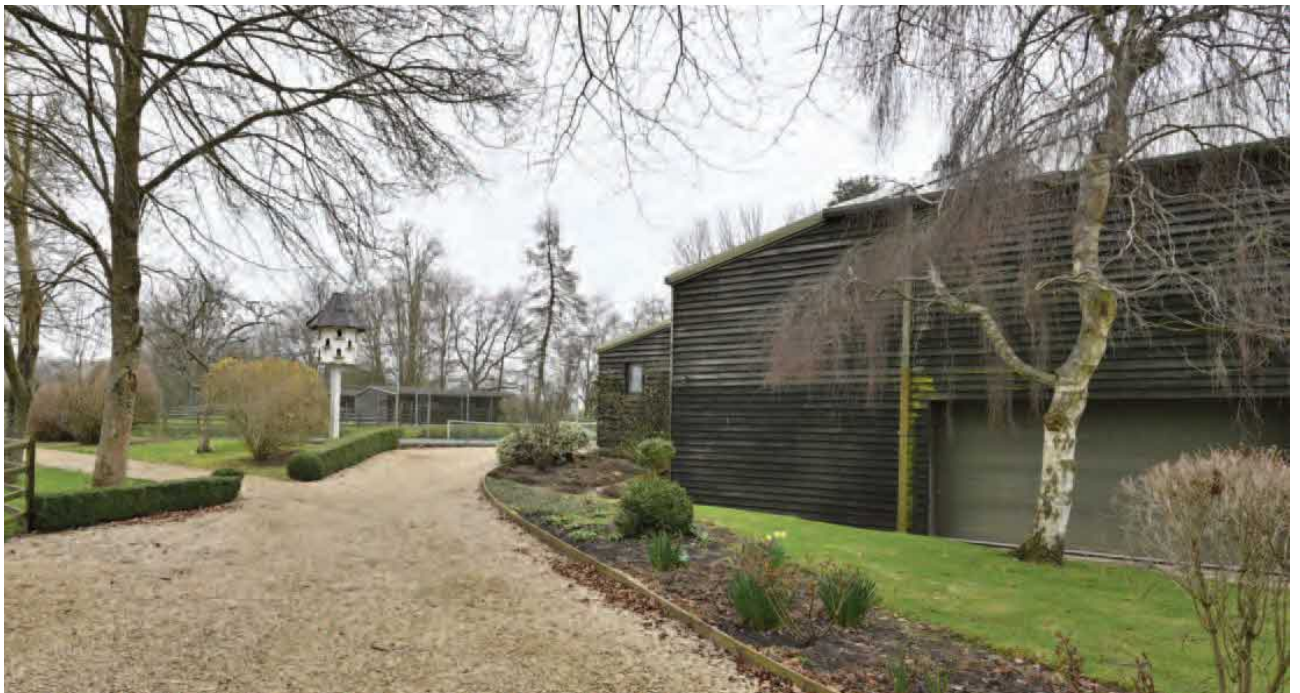
Fig. 11. The substantial and unsightly indoor riding arena dominates the north side of the site with additional stables, a manège and tennis courts extending westwards along the north side of the park.
