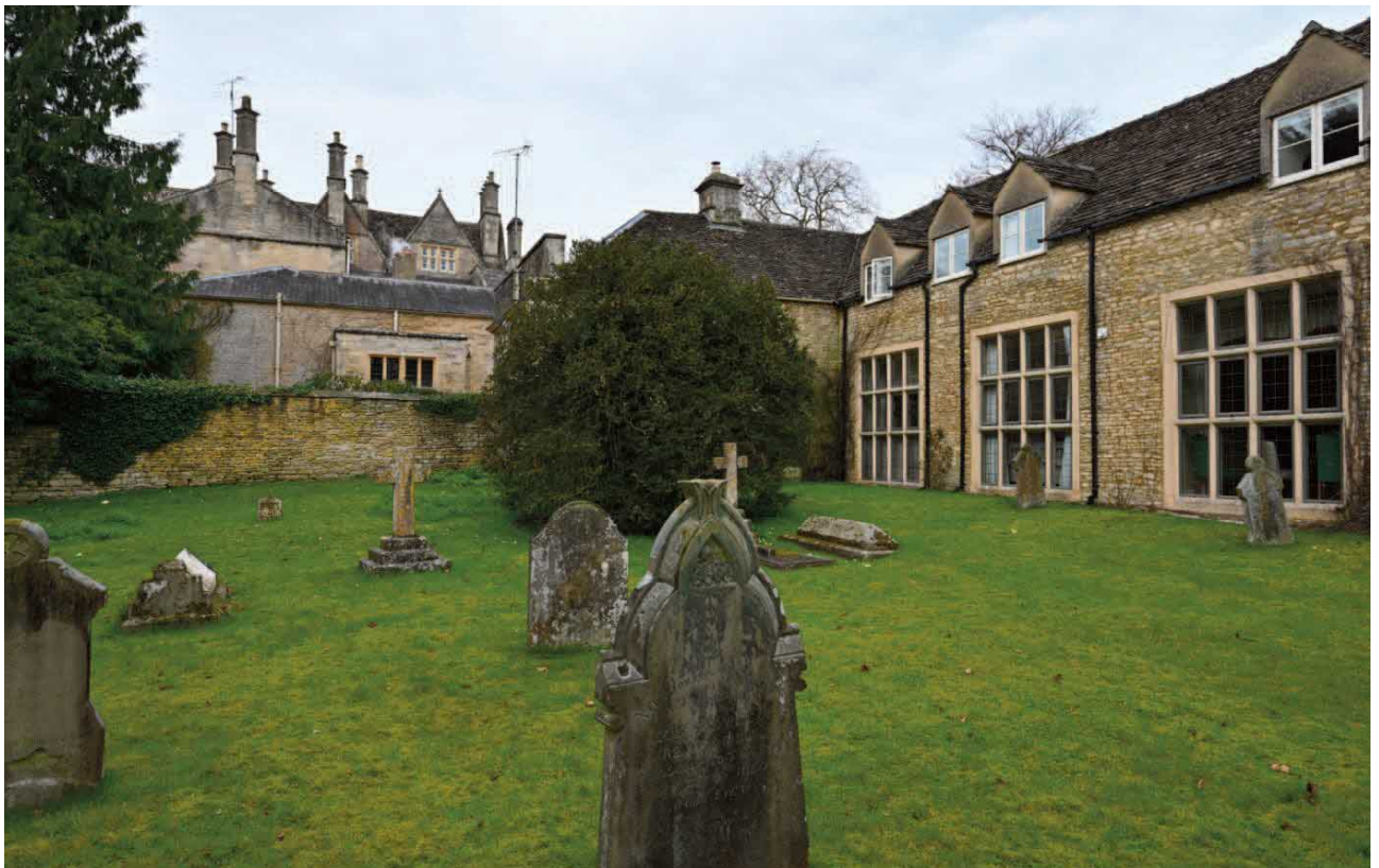
Fig. 7. The former stable and coach house range (barely recognizable after its 1980's conversion) overlooks the churchyard with the east elevation of Ampney Park visible on the left. The hipped single storey range is the former smoking room and ballroom extension now a library and swimming pool with its entrance porch.
