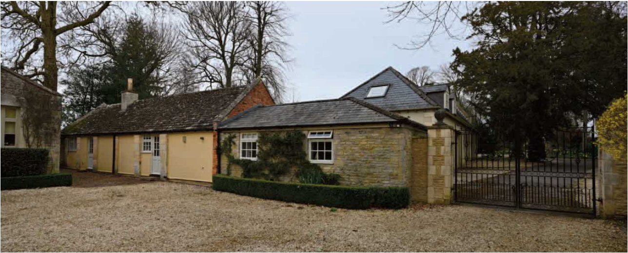
Fig 12. The historic former workshop and garden store (now converted to staff accommodation), together with the attached modern hipped range to the right, enclose the south side of the stable yard. The adjacent wall and gates enclosing the inner service yard are modern.
