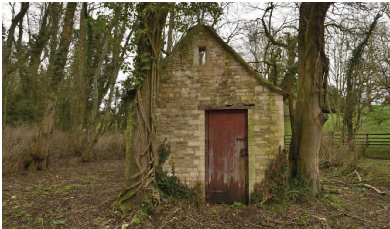
Fig. 30. The east pump house has a raised block for an early electrically driven engine doubtless used for pumping water up to the main house,. The absence of other fuel sources
