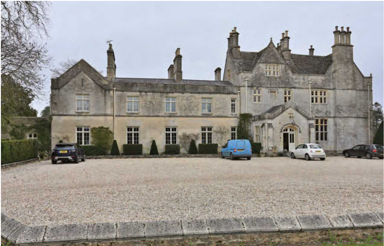
Fig. 16. The west front with the taller early 17th century principal range on the right and the early 19th century north range on the left. A single storey 19th century parapeted lean-to range is just visible to the left.
