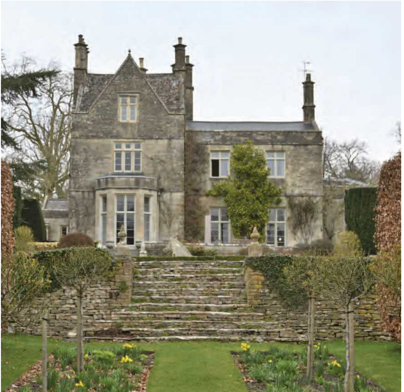
Fig. 17. The south elevation of the 17th century principal range is only one room wide, with its early 19th century east extension replacing the earlier extension shown set further back on the 1712 Kip drawing.
