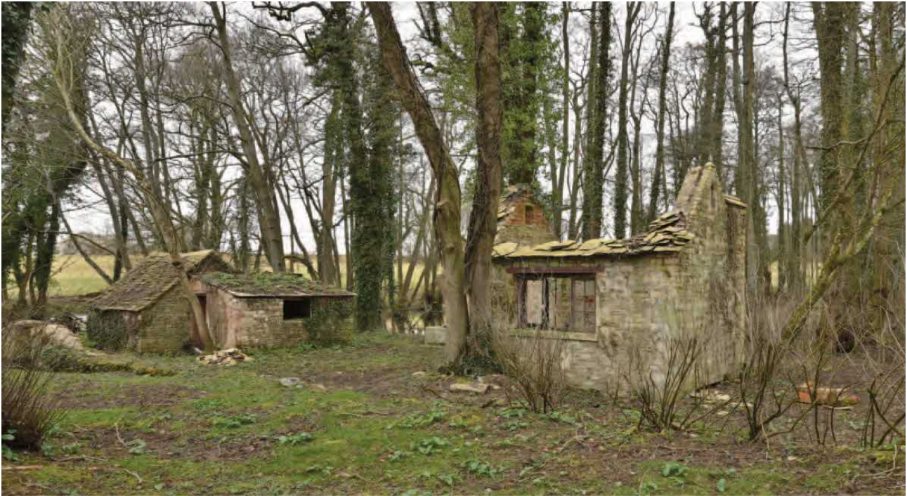
Fig. 27. The late 19th century pump house with its later brick lean-to extension and in the foreground the early 20th century pump house containing the engine bed mounting almost certainly for an electric pump.
