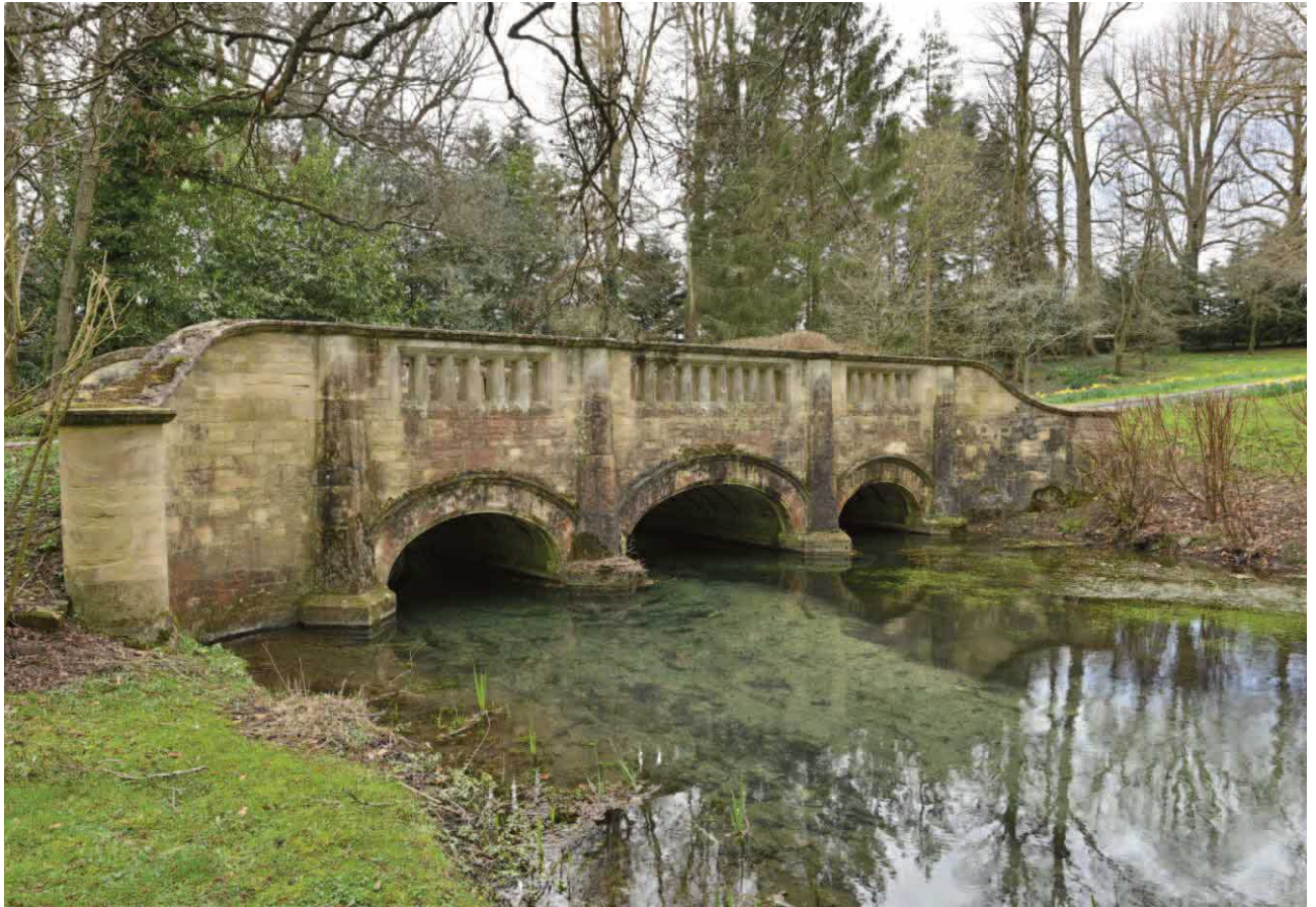
Fig. 25. The c.1902 bridge carrying the west drive over the Ampney Brook. The bridge is screened from views to the house by the parkland planting to either side of the brook and the intervening rising ground. This wooded area is accessed from the Park across a timber clapper bridge. It comprises an area of marshland enclosed within the open woodland and contains a series of interconnected ponds and sluices, connected by narrow paths with stone clapper bridges and timber boarding over the sluices.
