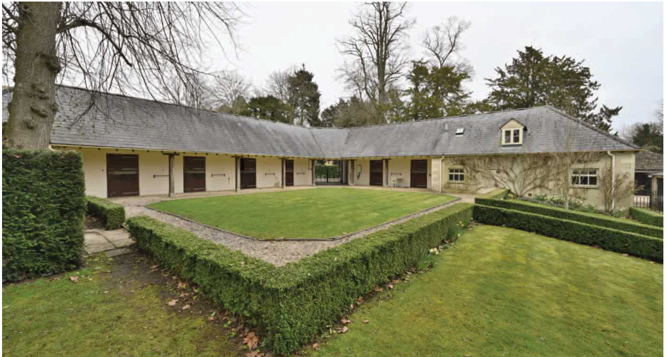
Fig. 10. The disused modern stable yard with the staff flat and garage range on the right. A historic range of workshops and staff accommodation on the south side of this yard (not shown) separates it from the house.
