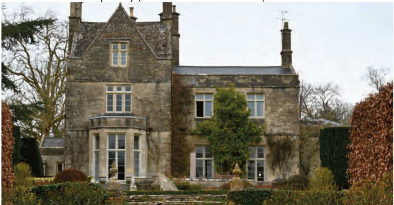
Fig.6. The south elevation with the mid-19th century two storey extension and the single storey late 19th century library or smoking room just visible on the right.
