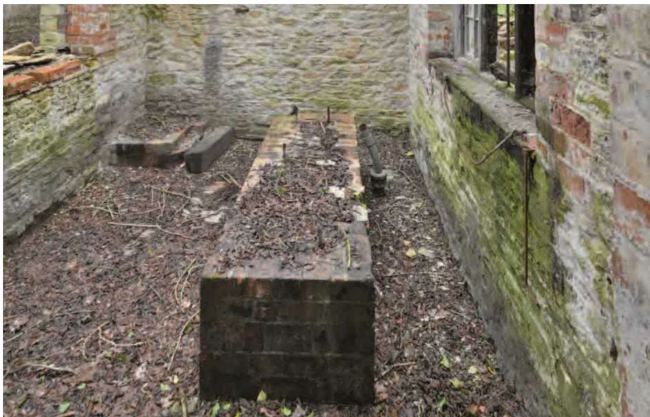
Fig. 31. The interior of the east pump house with the raised engine base and an associated water pipe.
