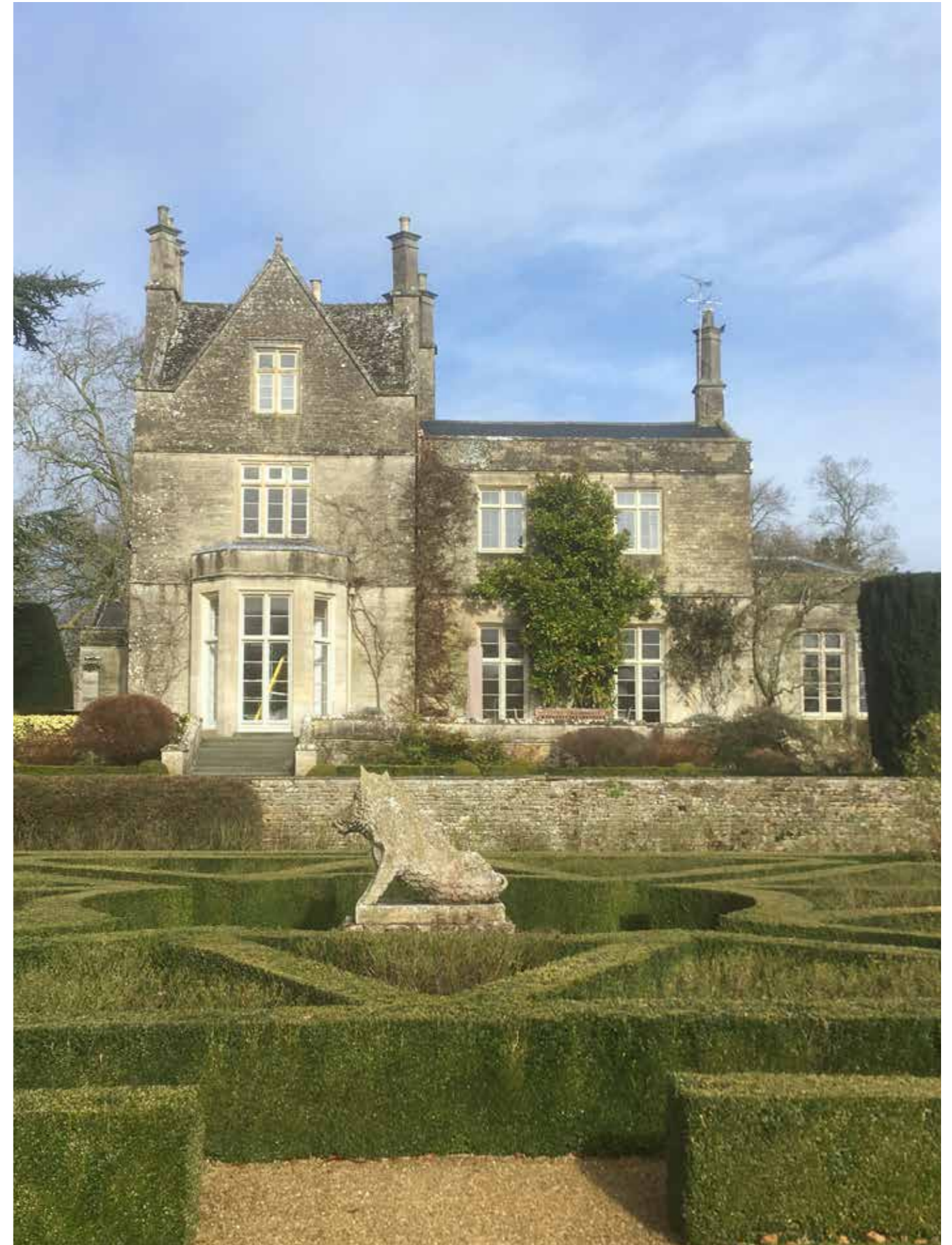
Photograph of Ampney Park south elevation at present
