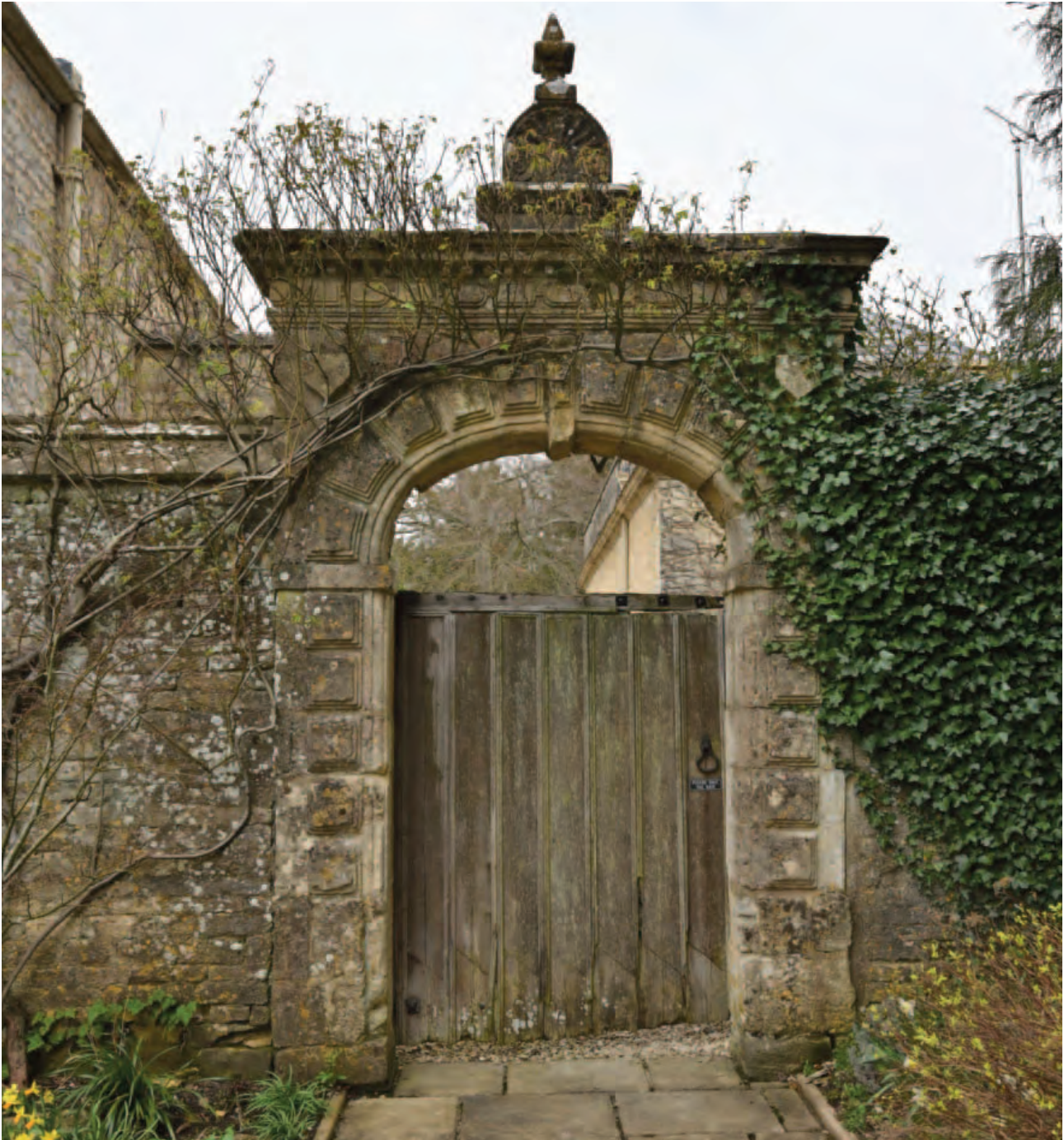
Fig. 18. The more ornate south face of the garden entrance gate. This may be the arched entrance shown on the Kip drawing at the entrance to the churchyard, which now has a simple gate set in the wall. The repair of this entrance gate has recently been granted listed building consent
