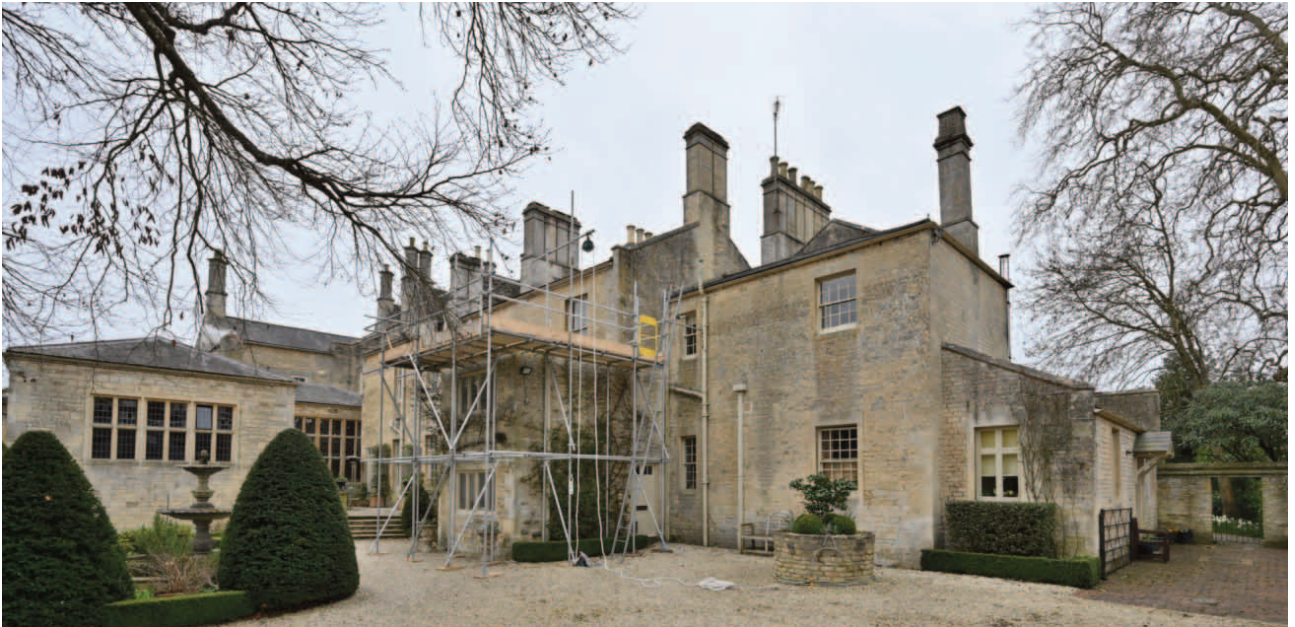
Fig. 19. The mansion seen from the north service yard with the early 20th century former ball room now a swimming pool on the left separated by a narrow courtyard from the early 19th century extension with the later 19th century hipped and parapeted cross wing at the north (righthand) end. The substantial late 19th century stone mullioned window lighting the billiard room can just be seen across the raised terrace and to the right of the house is an arched opening leading to the west front of the house.
