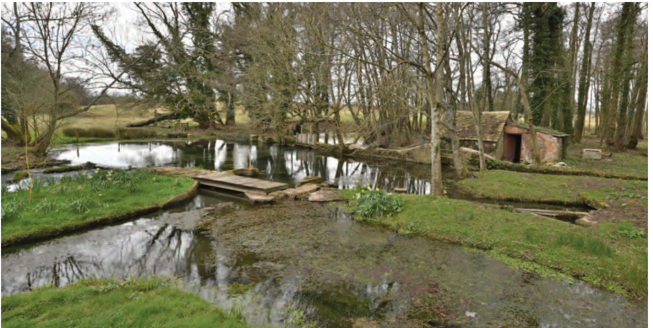
Fig. 26. The late 19th century west pump house with the sluices and reservoirs controlling the flow of water through the park in the foreground.
