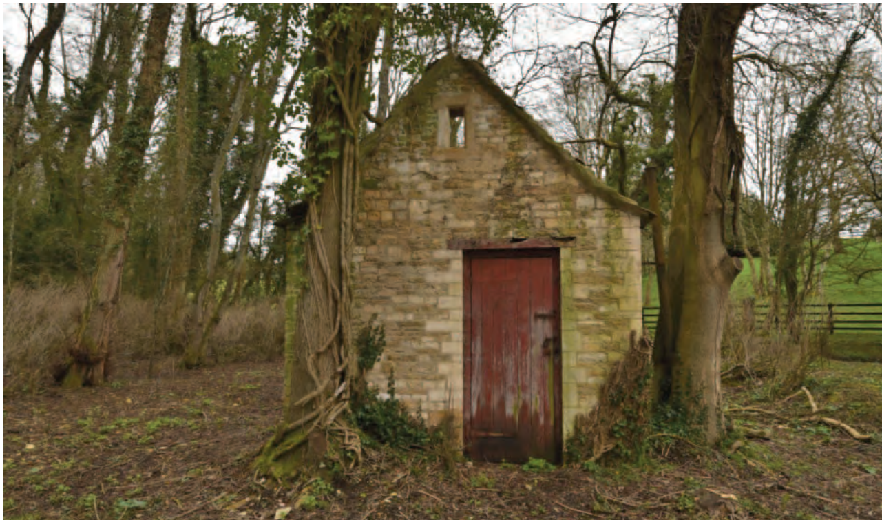
Fig. 30. The east pump house has a raised block for an early electrically driven engine doubtless used for pumping water up to the main house,. The absence of other fuel sources
