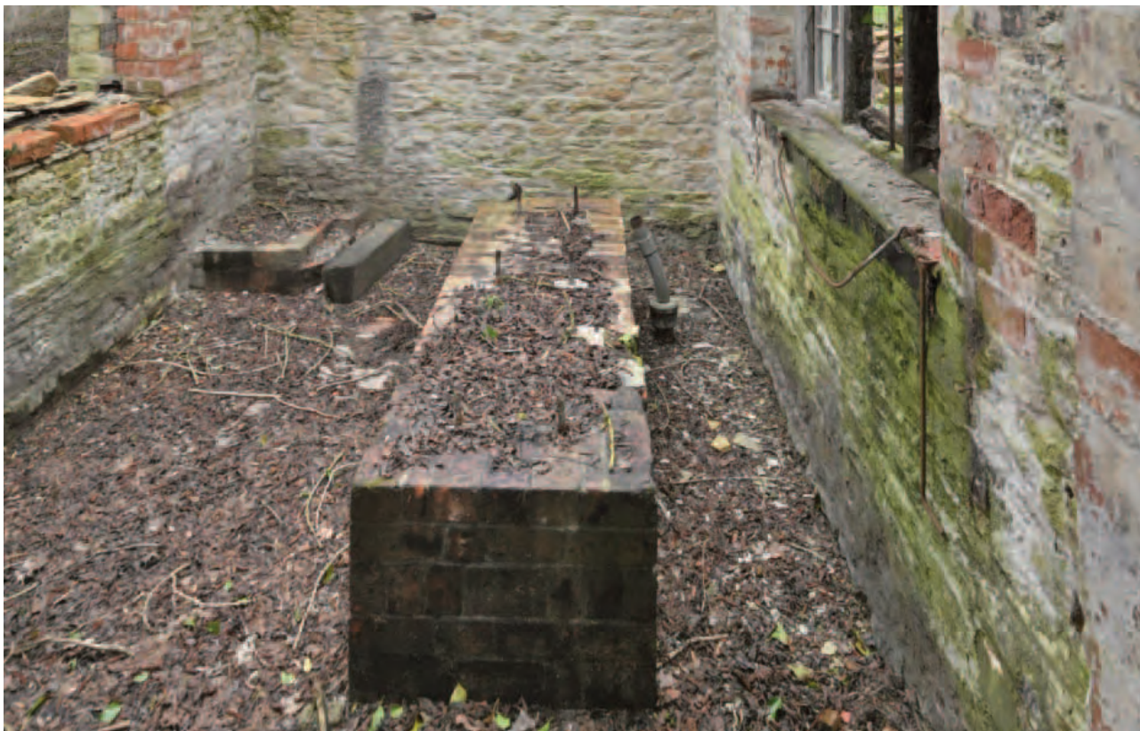
Fig. 31. The interior of the east pump house with the raised engine base and an associated water pipe.
