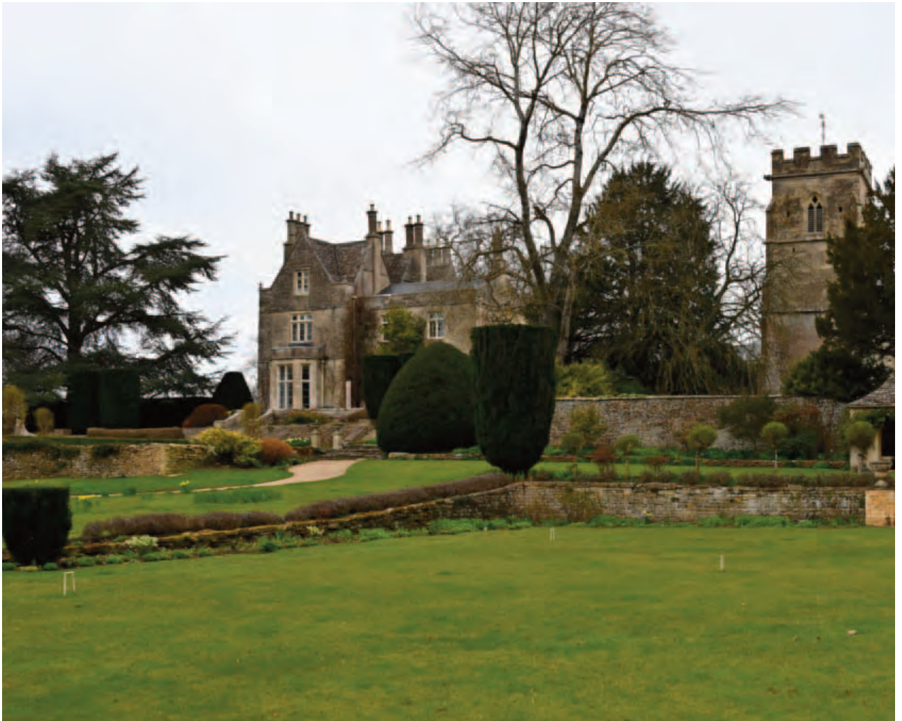
Fig 1. The current house, seen in its carefully landscaped grounds immediately adjacent to the parish church which dates back to Saxon times.
