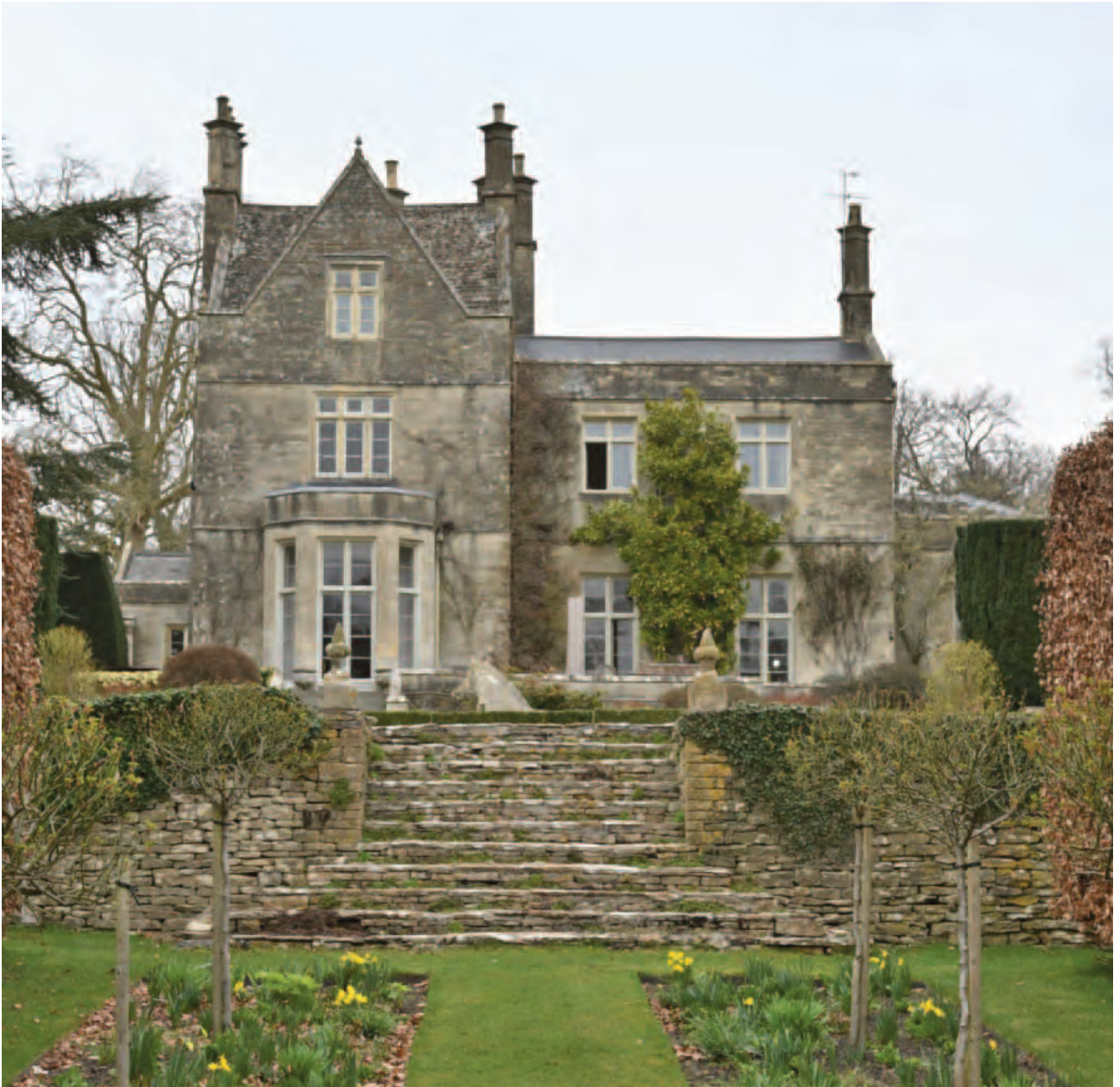
Fig. 17. The south elevation of the 17th century principal range is only one room wide, with its early 19th century east extension replacing the earlier extension shown set further back on the 1712 Kip drawing.
