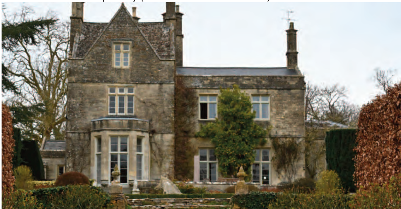
Fig.6. The south elevation with the mid-19th century two storey extension and the single storey late 19th century library or smoking room just visible on the right.
