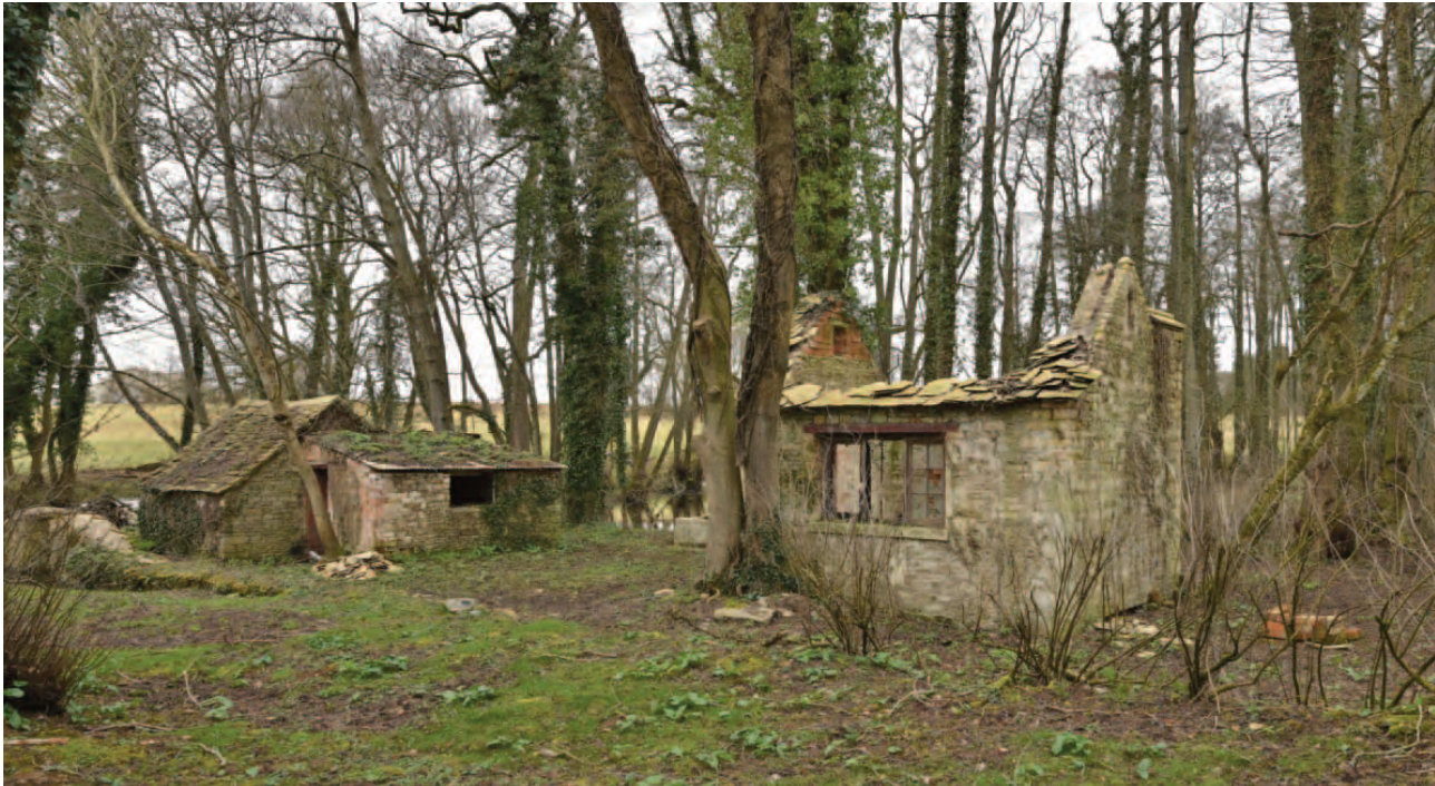
Fig. 27. The late 19th century pump house with its later brick lean-to extension and in the foreground the early 20th century pump house containing the engine bed mounting almost certainly for an electric pump.
