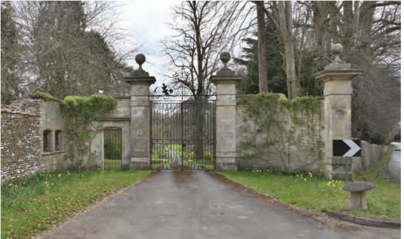
Fig. 22 The early 20th century (erected between 1902 - 1920) west entrance to the park with its asymmetrical form and stone rubble extension to the north wing wall (shown prior to repair of the collapsed section). The north wall continues westwards as a tall coursed rubble wall enclosing the open ground adjacent to the entrance, and limiting views towards woodland and pasture. A section of this wall has recently been rebuilt following vehicle impact damage. At the west end, the wall is separated from the road by a field gate opening onto a wooded track.
