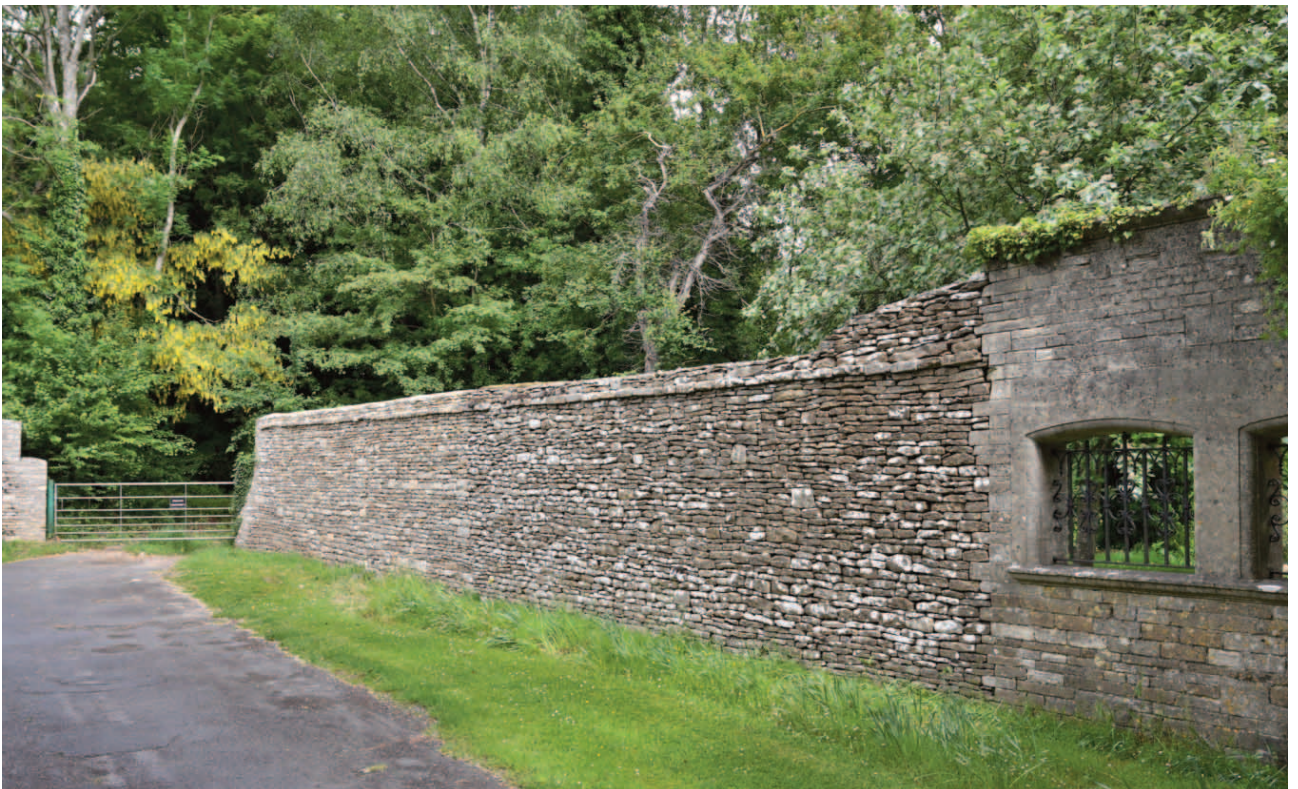
Fig. 23. Detail of the north wing wall showing the rebuilt section at its northern end adjacent to the private gated access to land outside the ownership of Ampney Park.
