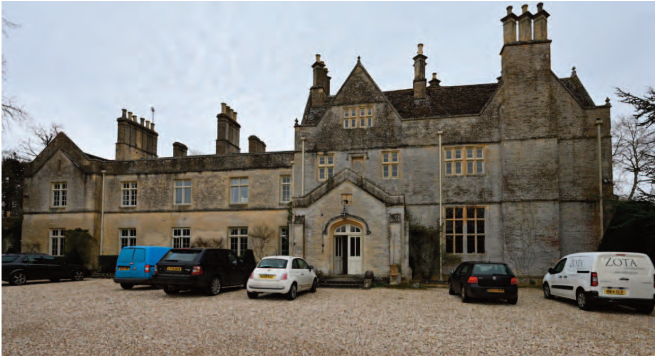
Fig 5. The taller 17th century principal range on the right with the early 19th century double pile north range on the left terminating in a short later 19th century cross wing.
