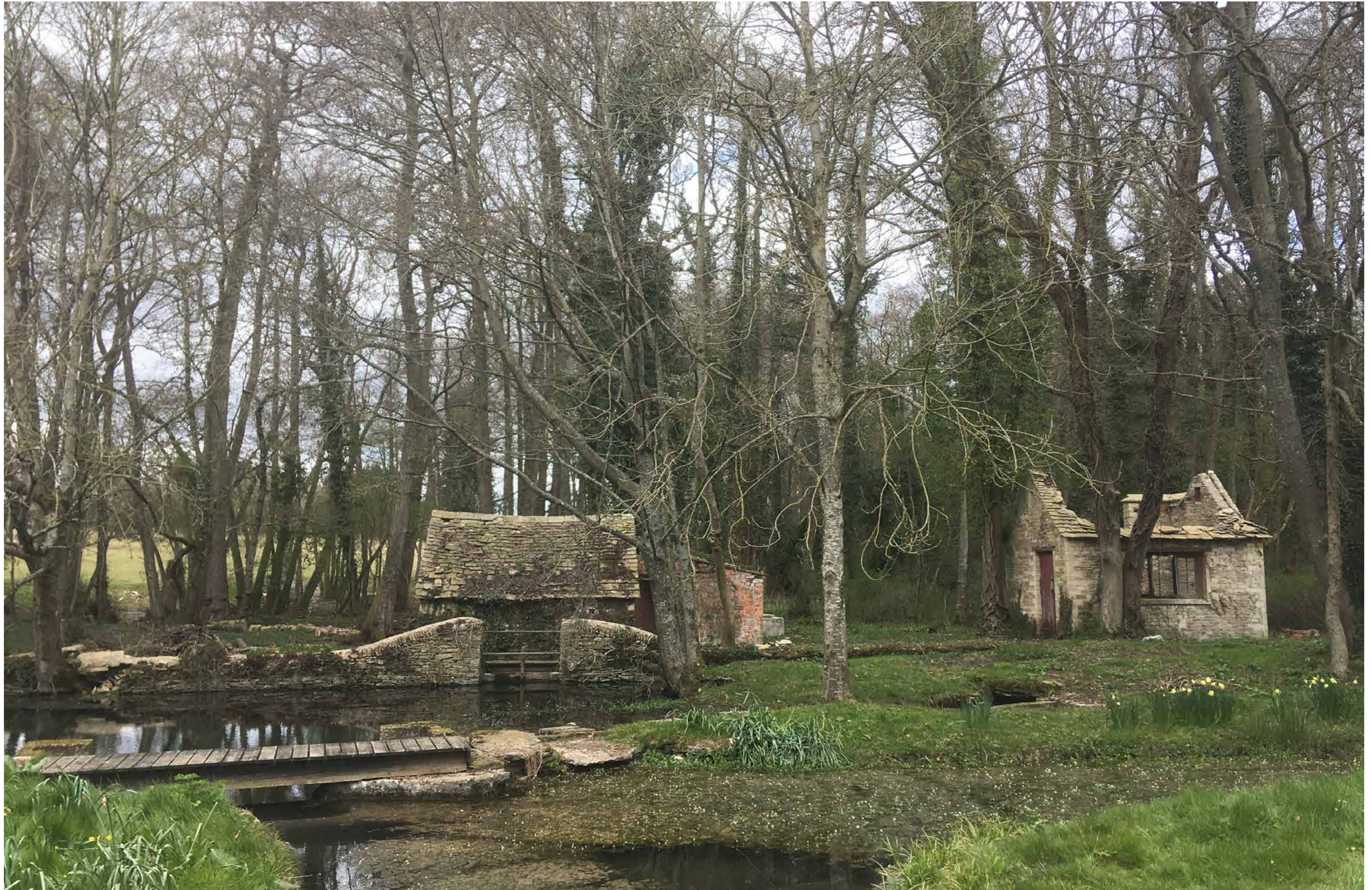
Photograph of the Listed Pumpouses from Winterwell
