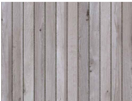
Weathered timber cladding
