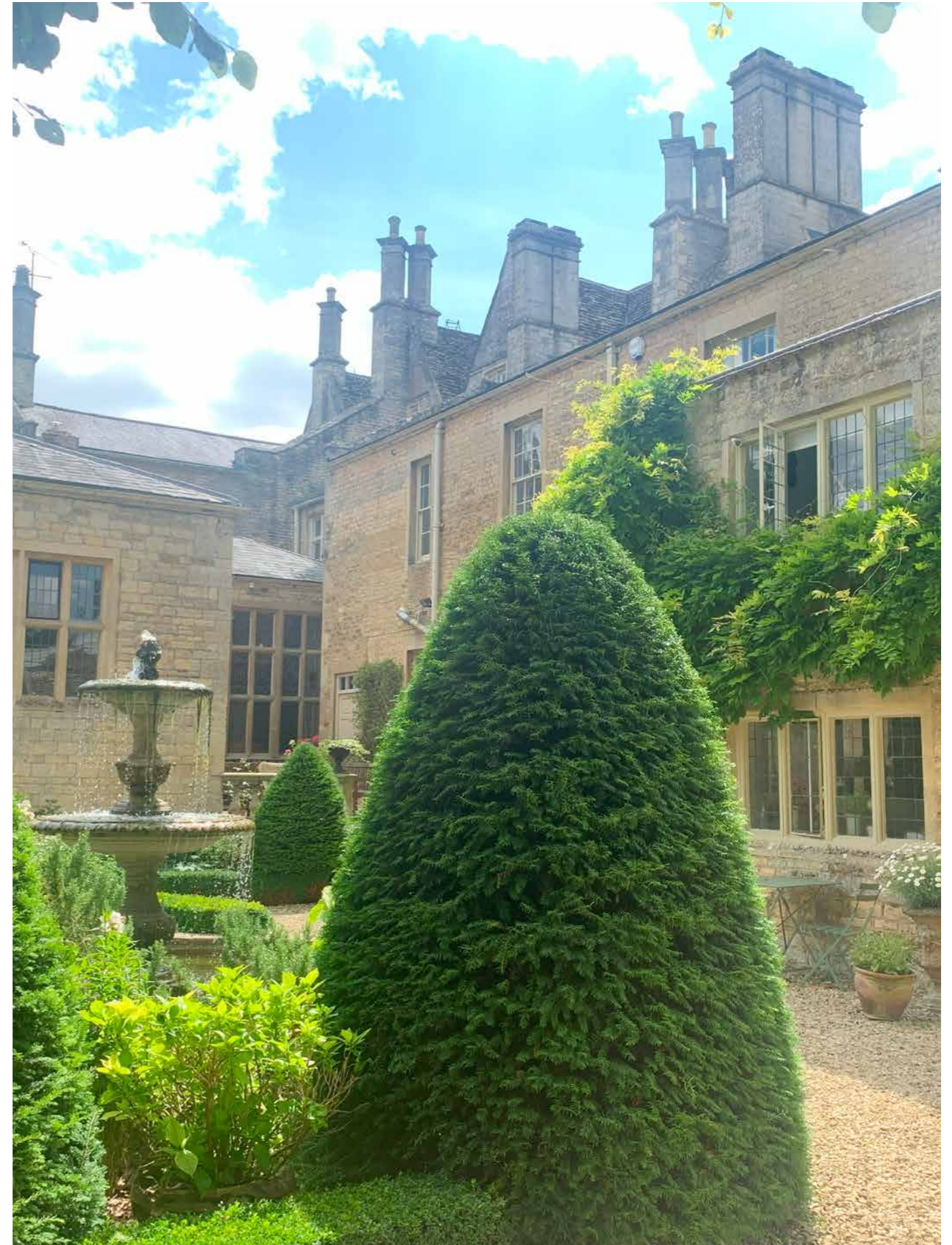
Photograph of Ampney Park rear courtyard
