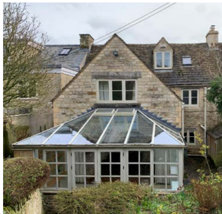
Existing Rear Conservatory
