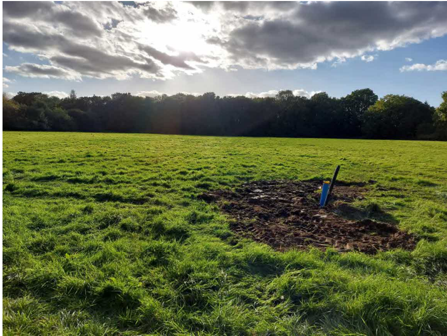
Plate 7 – Pipework installed in TP1 for BRE365 Soakage test.
