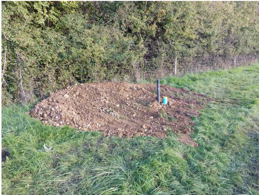
Plate 10 – Trial pit TP2 arisings and pipework installed for BRE365 Soakage test.
