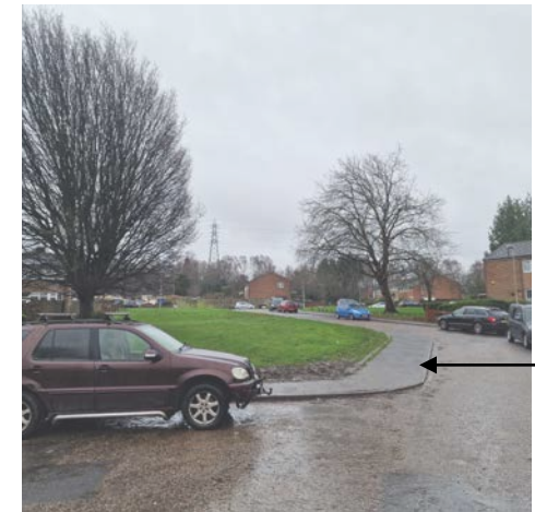
Informal parking occurring along Redhorn Close and at the turning head
