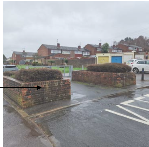
Traffic calming measure between Russell Gardens and Fitzworth Avenue.
