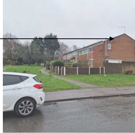
2 Story terraced dwellings to the south of the site. Buff Brick and gabled ended roofs.
