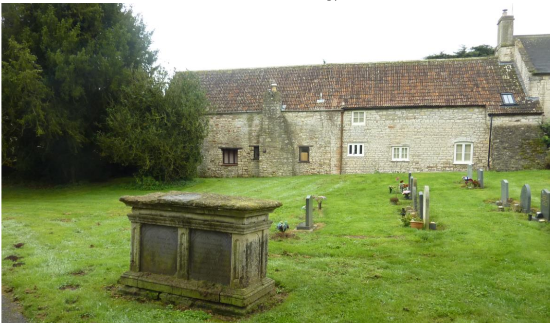
Figure 3 – Rear elevation of Kilmersdon Meeting Room and part of Orange Farmhouse
