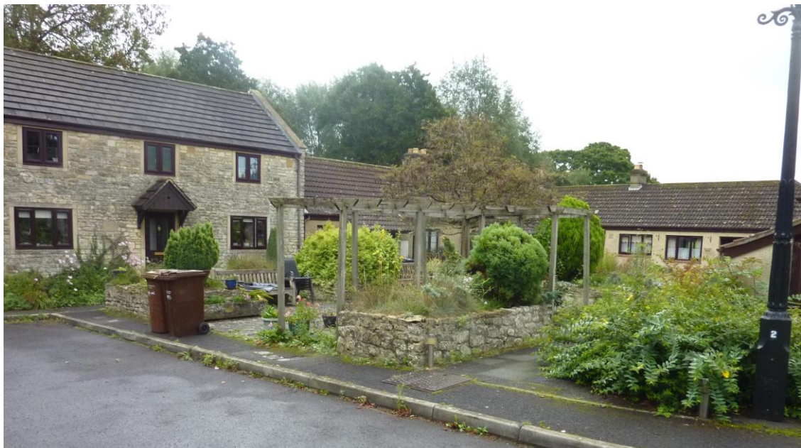
Figure 9 – Central courtyard garden in Coles Garden housing
