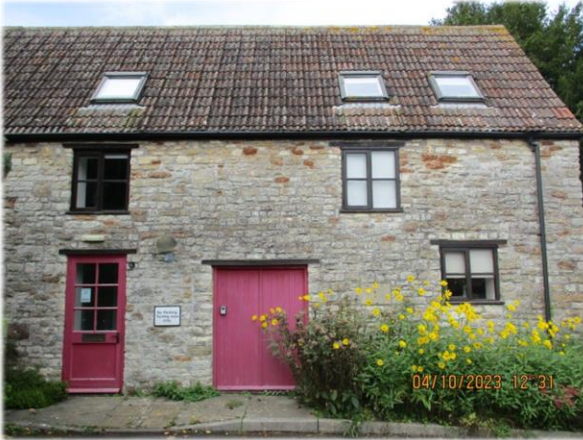
Front, southeast-facing building elevation (left) with one missing roof tile to immediate right of roof window (right)
