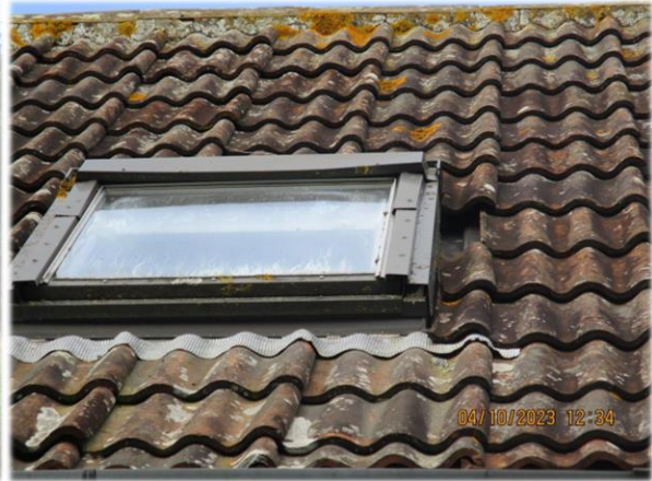
Front, southeast-facing building elevation (left) with one missing roof tile to immediate right of roof window (right)
